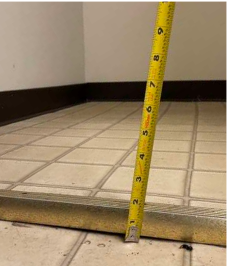
Men’s Restroom Floor
