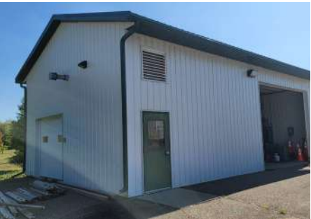
UV/Storage Building Exterior
