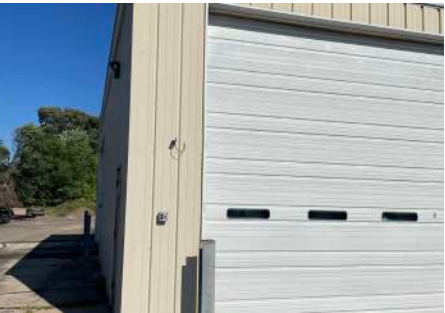
Metal Panel/South Corner
