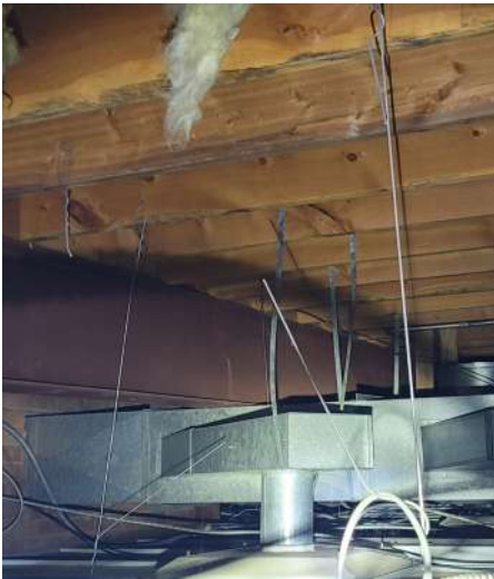
Roof Structural Support Members
