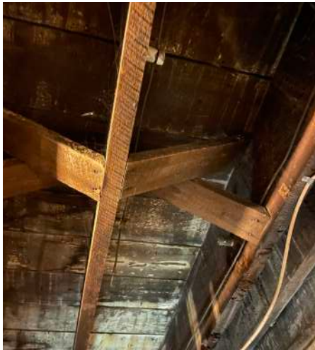
Subflooring Original Bank
