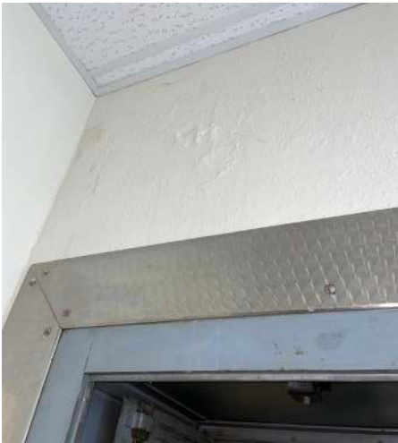
Village Hall Plaster Walls
