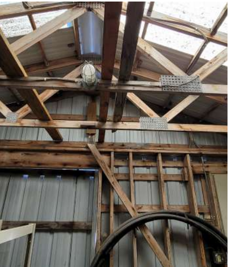
Animal Shelter Roof Trusses
