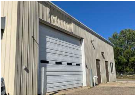
Metal Panel/Northern East Wall
