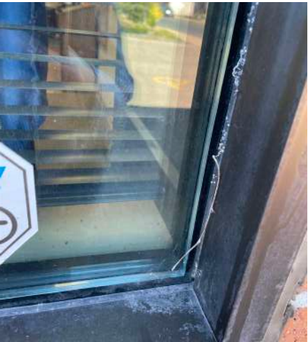
Seal at North Fixed Window
