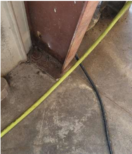
808 Building PEMB Frames
