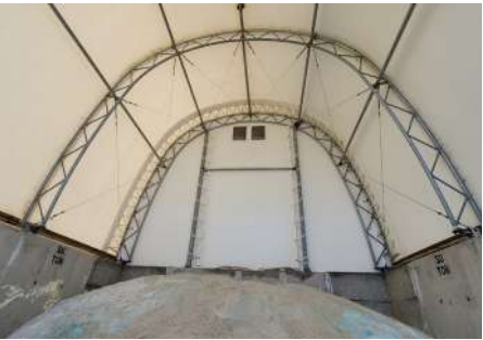
Hoop Structure/Salt Storage Roof
