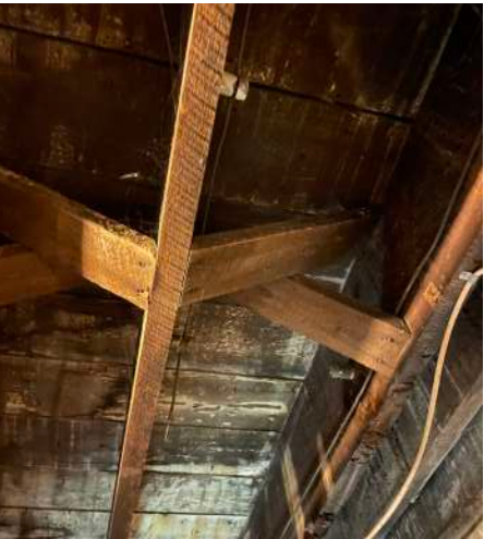
Subflooring Original Bank
