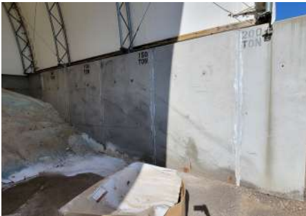
Hoop Structure/Salt Storage Wall
