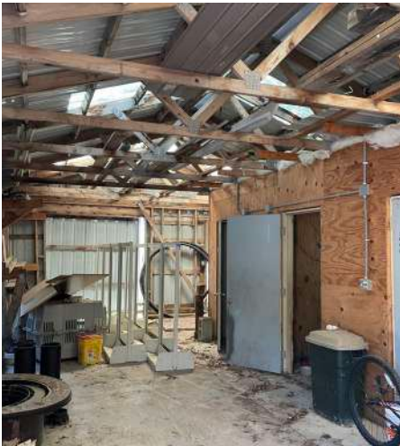
Interior Cold Storage Garage
