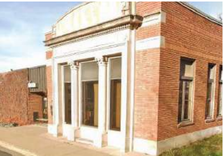
Exterior Facade Southeast Side
