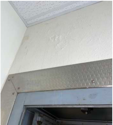
Village Hall Plaster Walls
