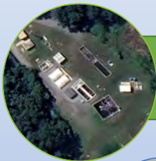
Hyde Park, NY - $3.5M WWTP Upgrade
