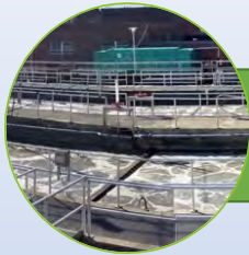
Kingston, NY - $10.2M WWTP Upgrade
