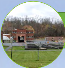
Beacon, NY - $5.9M WWTP Upgrade
