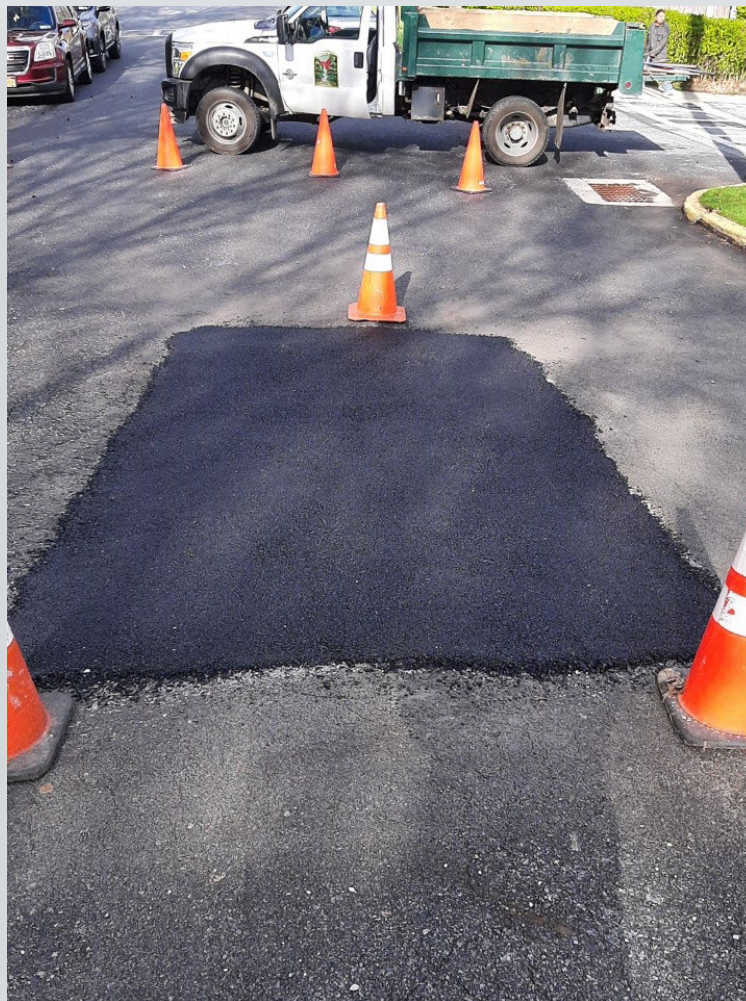
Merritt Ave - After
