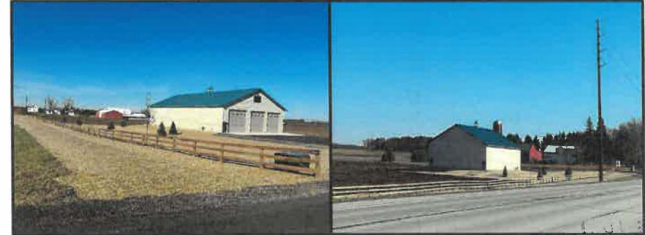
Lyons Storage Building, Burlington, WI
