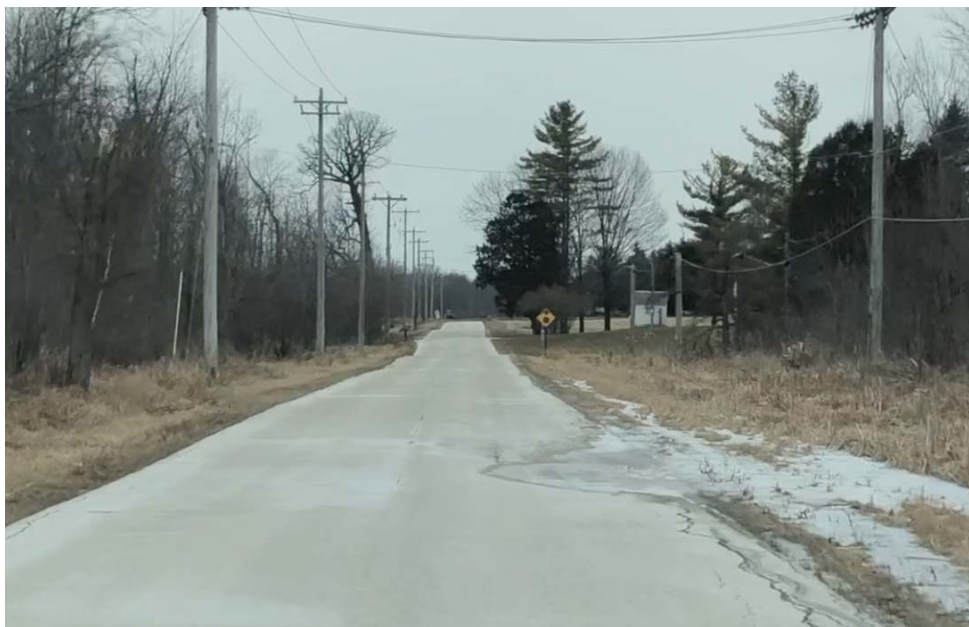
Overtopping and Ice on Roadway
