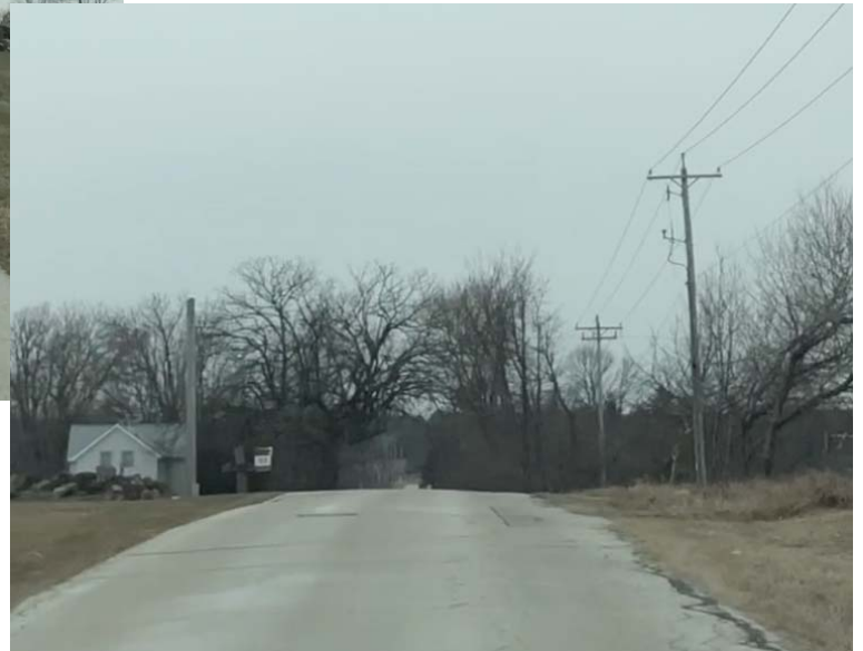
Substandard Vertical Curve Looking East
