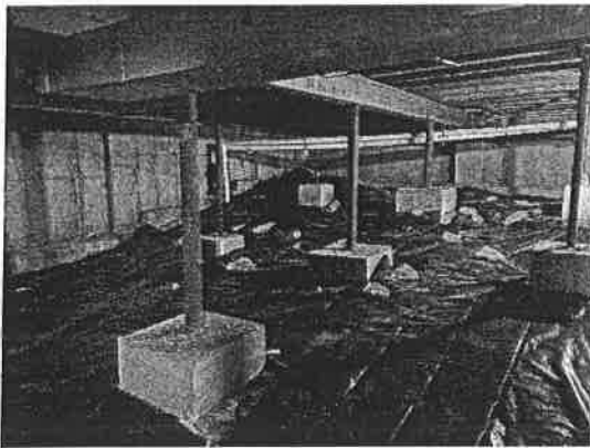
Photo 9 – Foundations and Wood Framing
