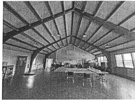
Photo 12 – Glulam Frames, Roof Joists
