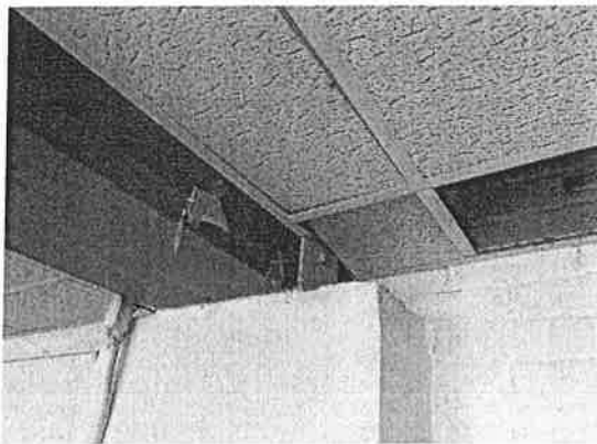
Photo 11 – Glulam on Pilaster
