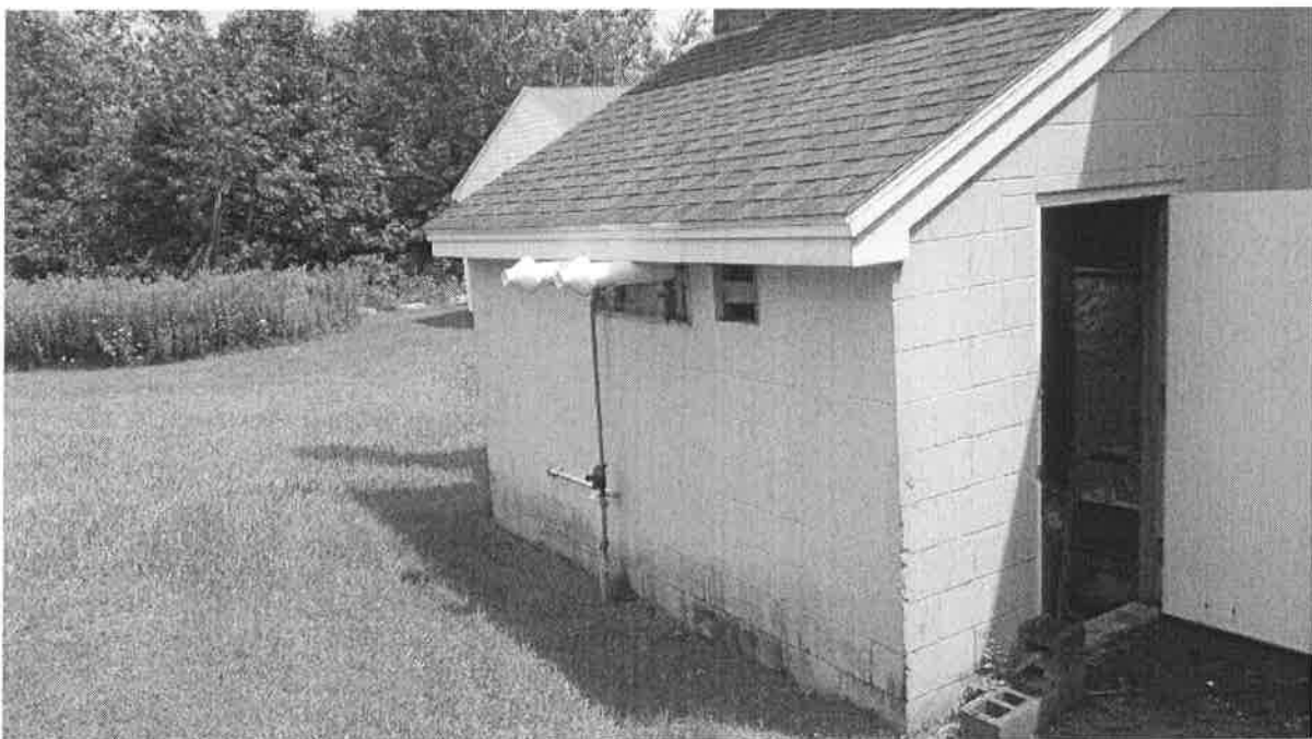
South AHU shed that contains two furnaces/AHUs
