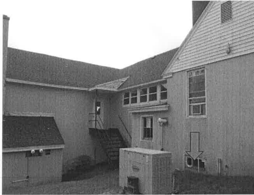
Exterior view of cellar window, (blue arrow pointing to plastic tube in window)
