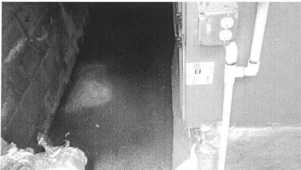
Moistened cement floor of east furnace shed
