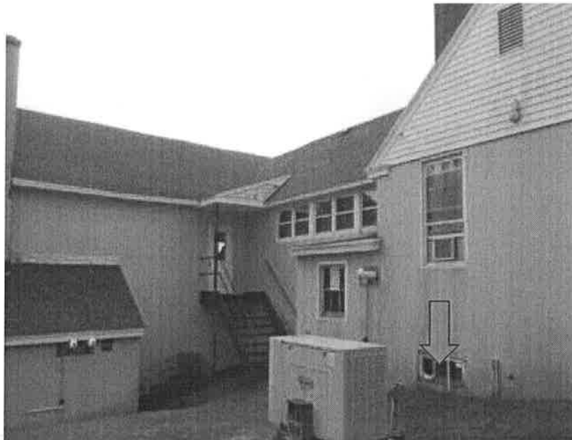
Exterior view of cellar window, (blue arrow pointing to plastic tube in window)
