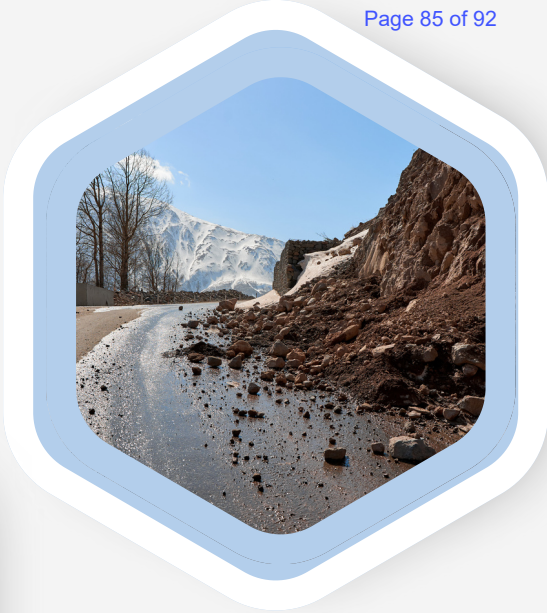
Landslide/ Slope Failure
