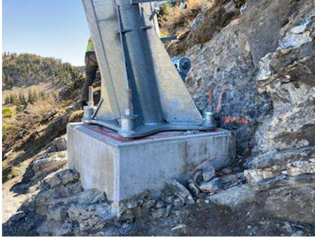
Completed Wyssen footing
