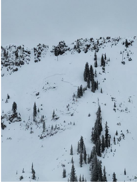
East Castle Wyssen installation (two towers visible)
