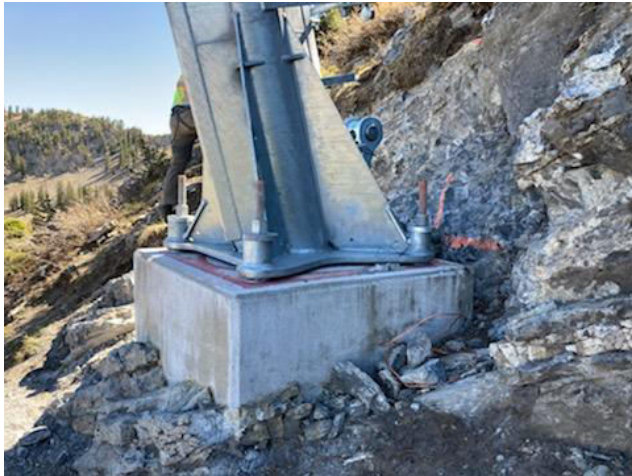
Completed Wyssen footing
