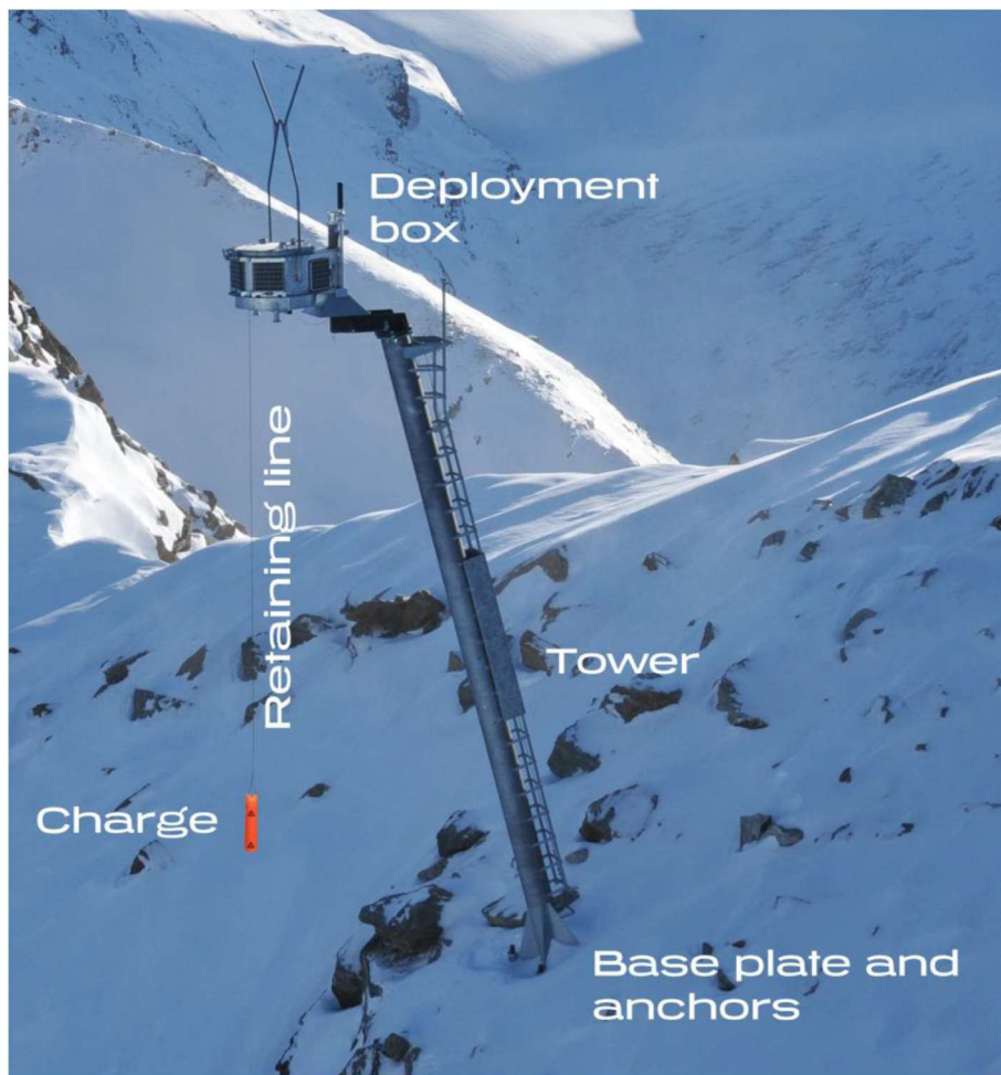
Figure 1 – Wyssen Tower with Deployment Box
