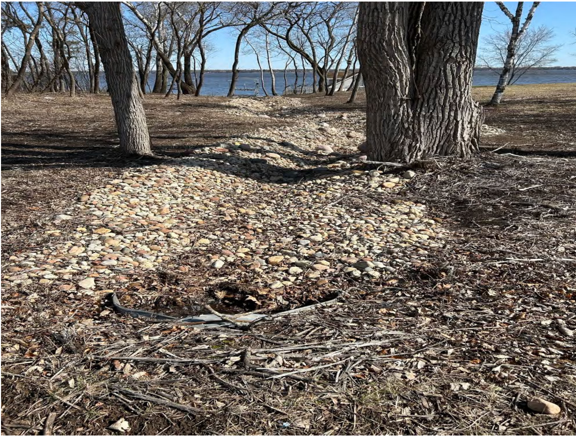
4404 Bellhaven drainage way photos:
