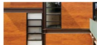
Wood paneling in storefront
