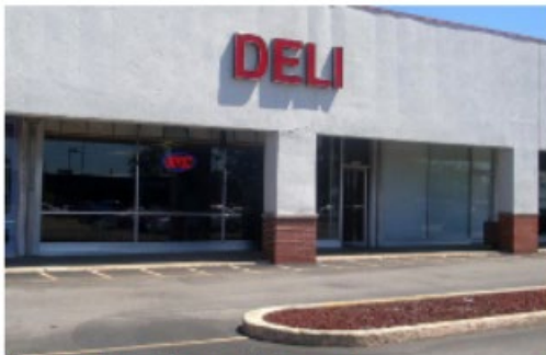
Unacceptable Signage Placement
