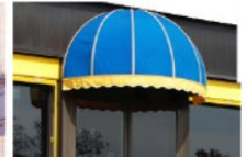
Example of Unacceptable Awning
