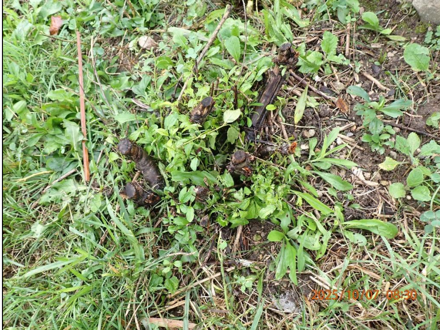
Waterville Dam Stump On Right Upstream Embankment 0022110072511.JPG
