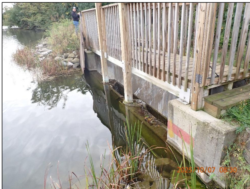
Waterville Dam Dam From Right Embankment 0022110072502.JPG
