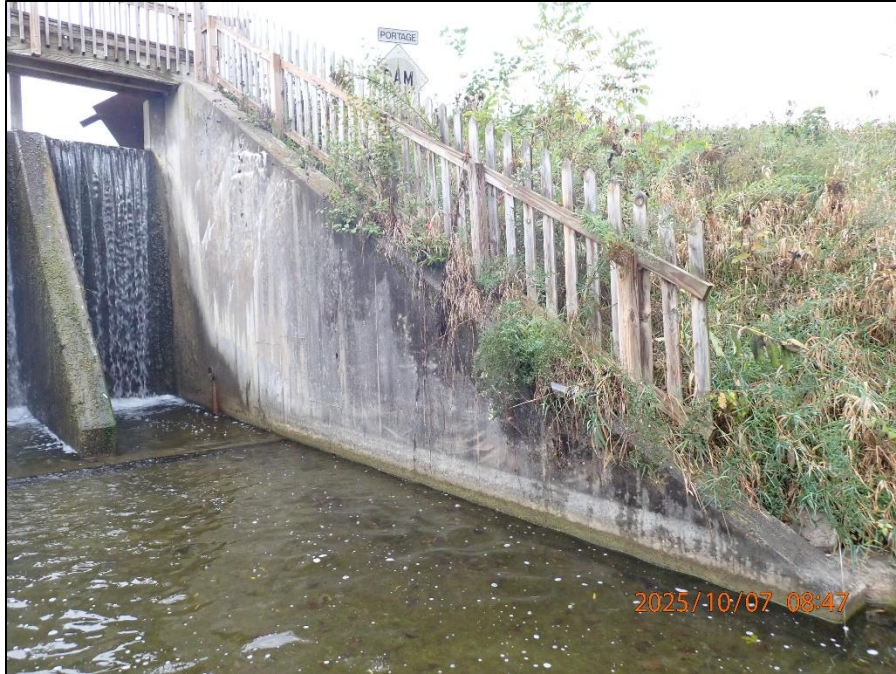
Waterville Dam Left Downstream Abutment 0022110072507.JPG
