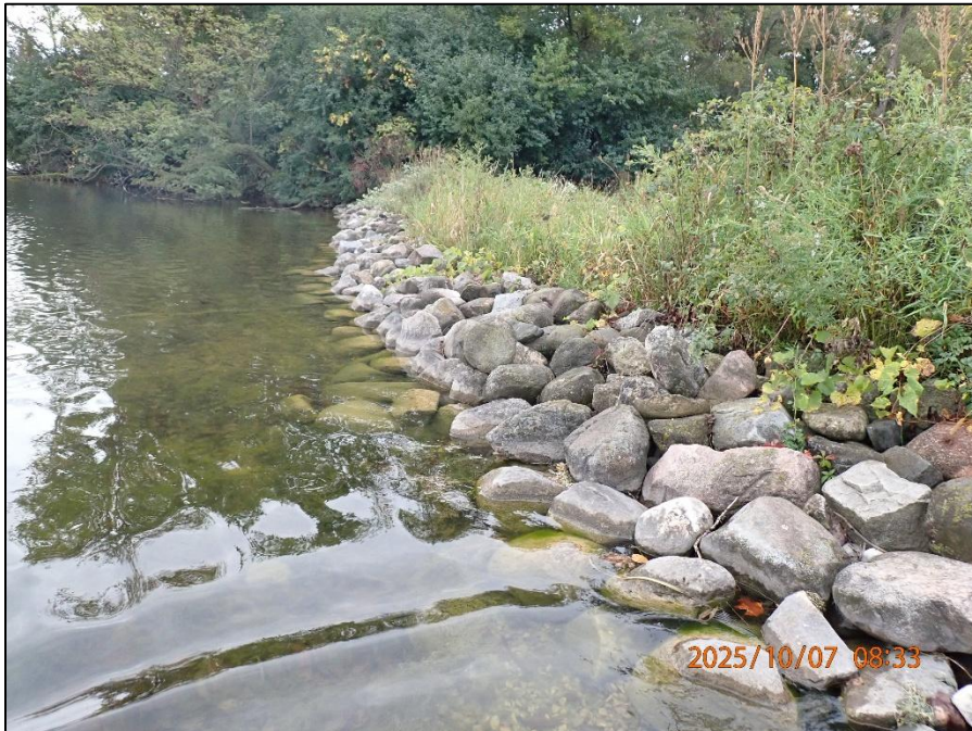
Waterville Dam Left Upstream Embankment 0022110072512.JPG
