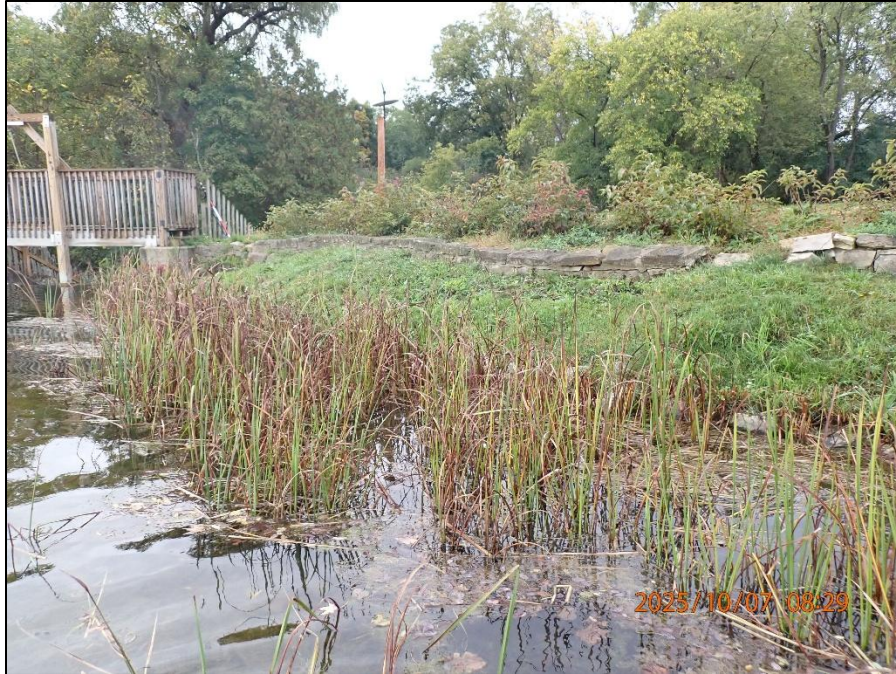
Waterville Dam Right Upstream Embankment 0022110072509.JPG
