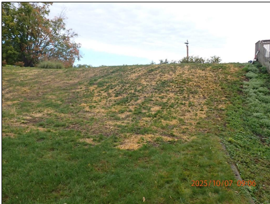
Waterville Dam Right Downstream Embankment 0022110072510.JPG
