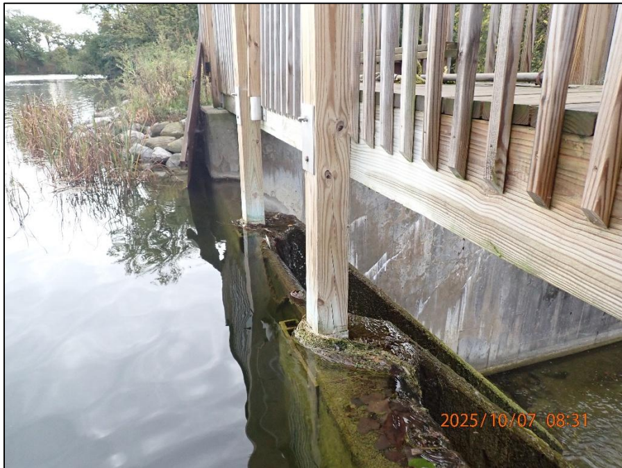
Waterville Dam Left Upstream Abutment 0022110072506.JPG
