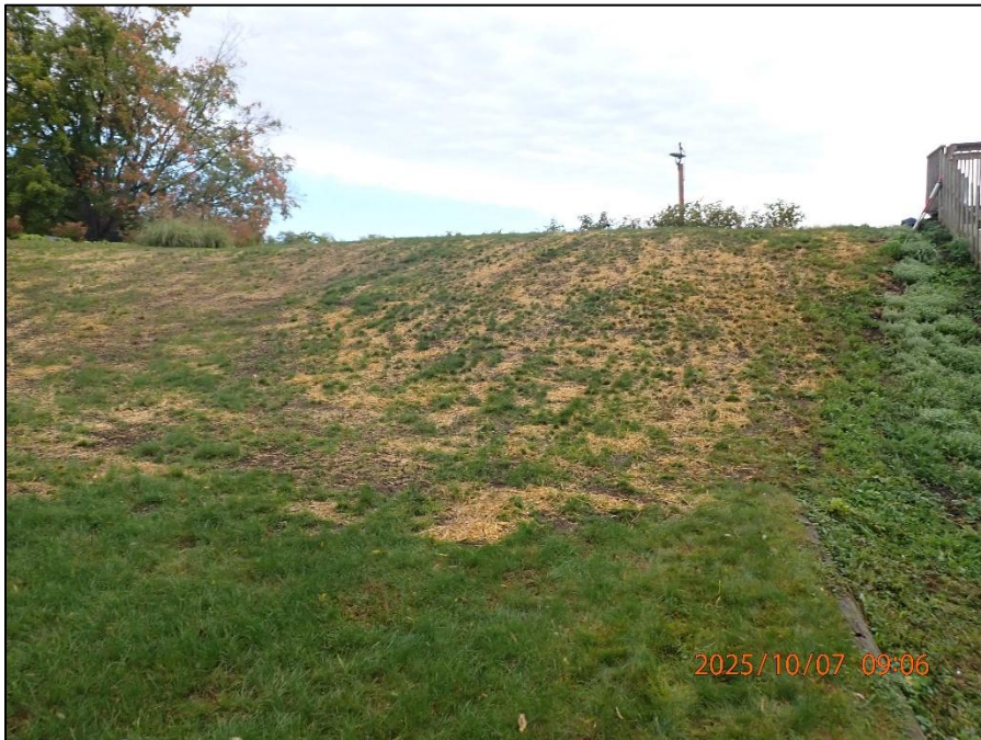
Waterville Dam Right Downstream Embankment 0022110072510.JPG
