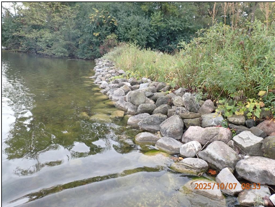
Waterville Dam Left Upstream Embankment 0022110072512.JPG
