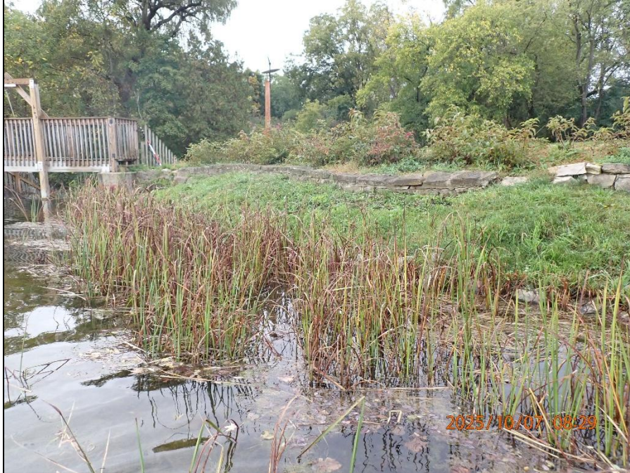
Waterville Dam Right Upstream Embankment 0022110072509.JPG
