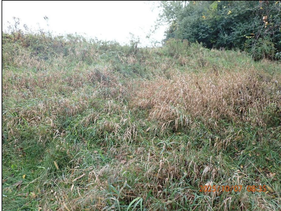
Waterville Dam Left Downstream Embankment 0022110072513.JPG
