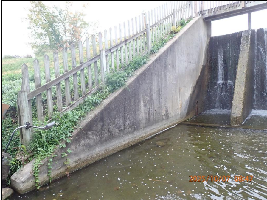
Waterville Dam Right Downstream Abutment 0022110072505.JPG
