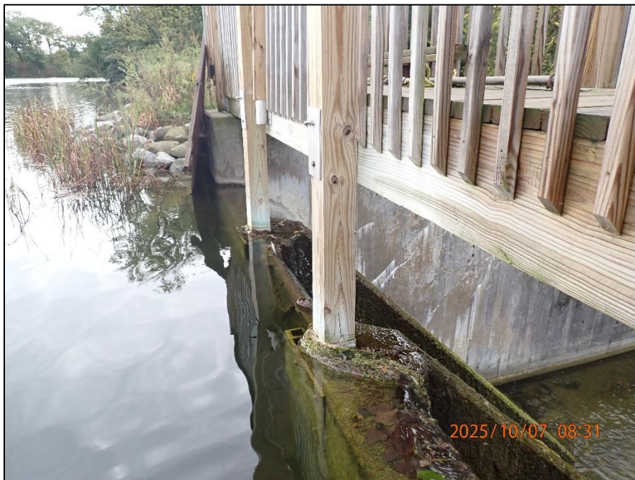
Waterville Dam Left Upstream Abutment 0022110072506.JPG
