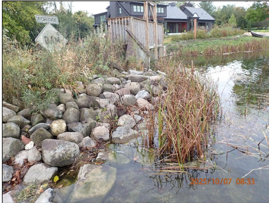
Waterville Dam Dam From Left Embankment 0022110072501.JPG
