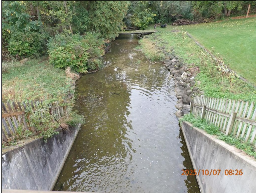
Waterville Dam Stream Downstream Of Dam 0022110072503.JPG
