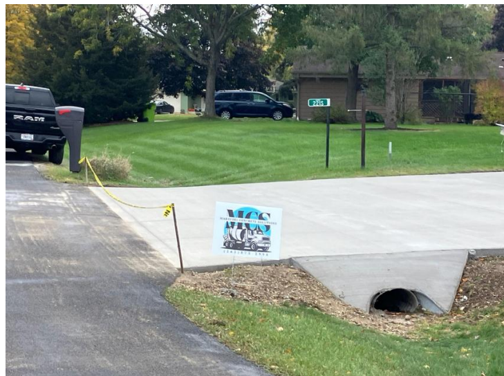
Photo: October 22, 2025 (newly poured driveway)
