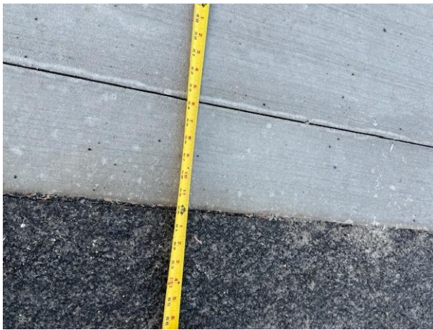
Image 1: 1 st joint (6" from edge of asphalt)
