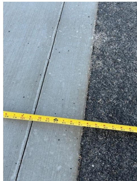
Image 4: Distance from 2 nd joint to asphalt
