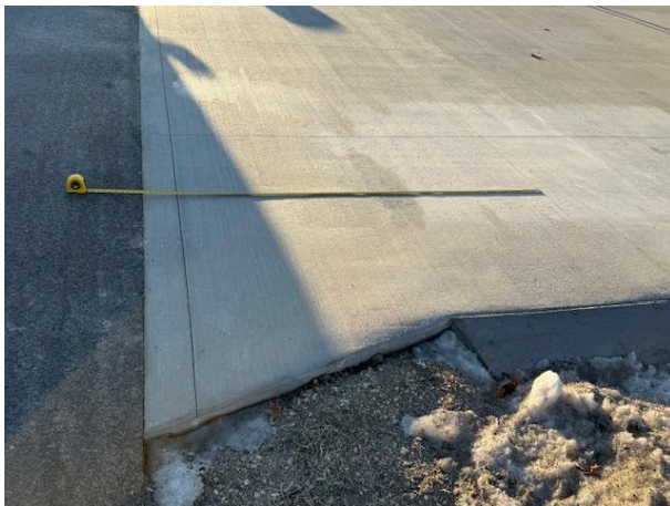
Image 3: 2 nd joint (7' 3" from edge of asphalt)
