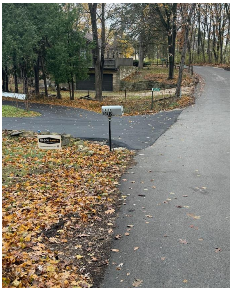
November 19, 2025 Photo (New Pavement)
