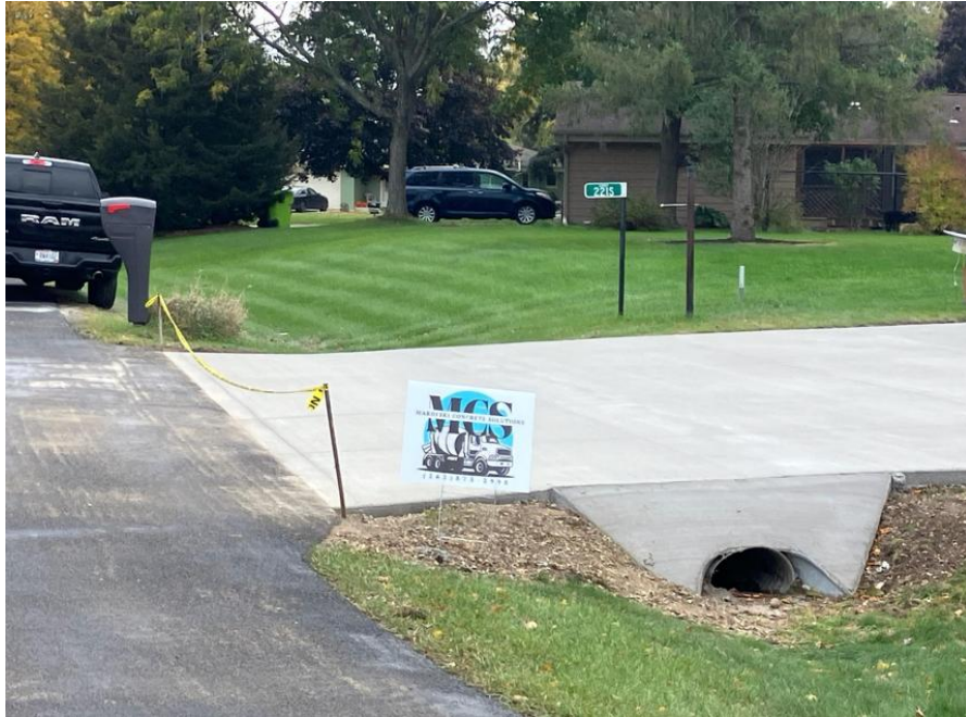
Photo: October 22, 2025 (newly poured driveway)
