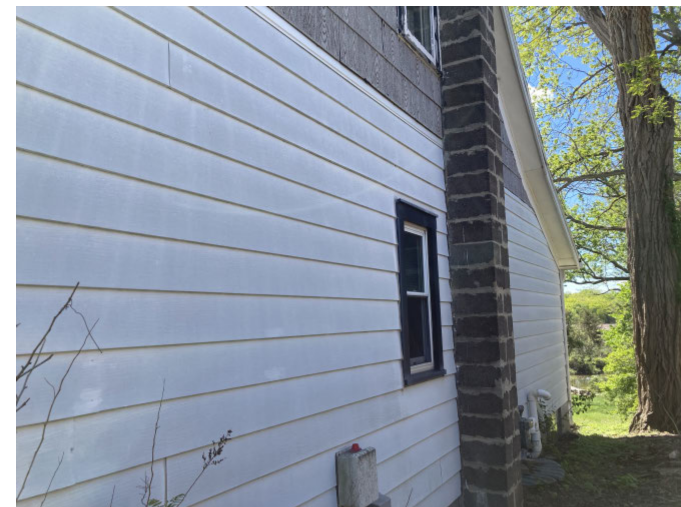
23 EXISTING EXTERIOR PHOTO - 9 3/8" = 1'-0"
