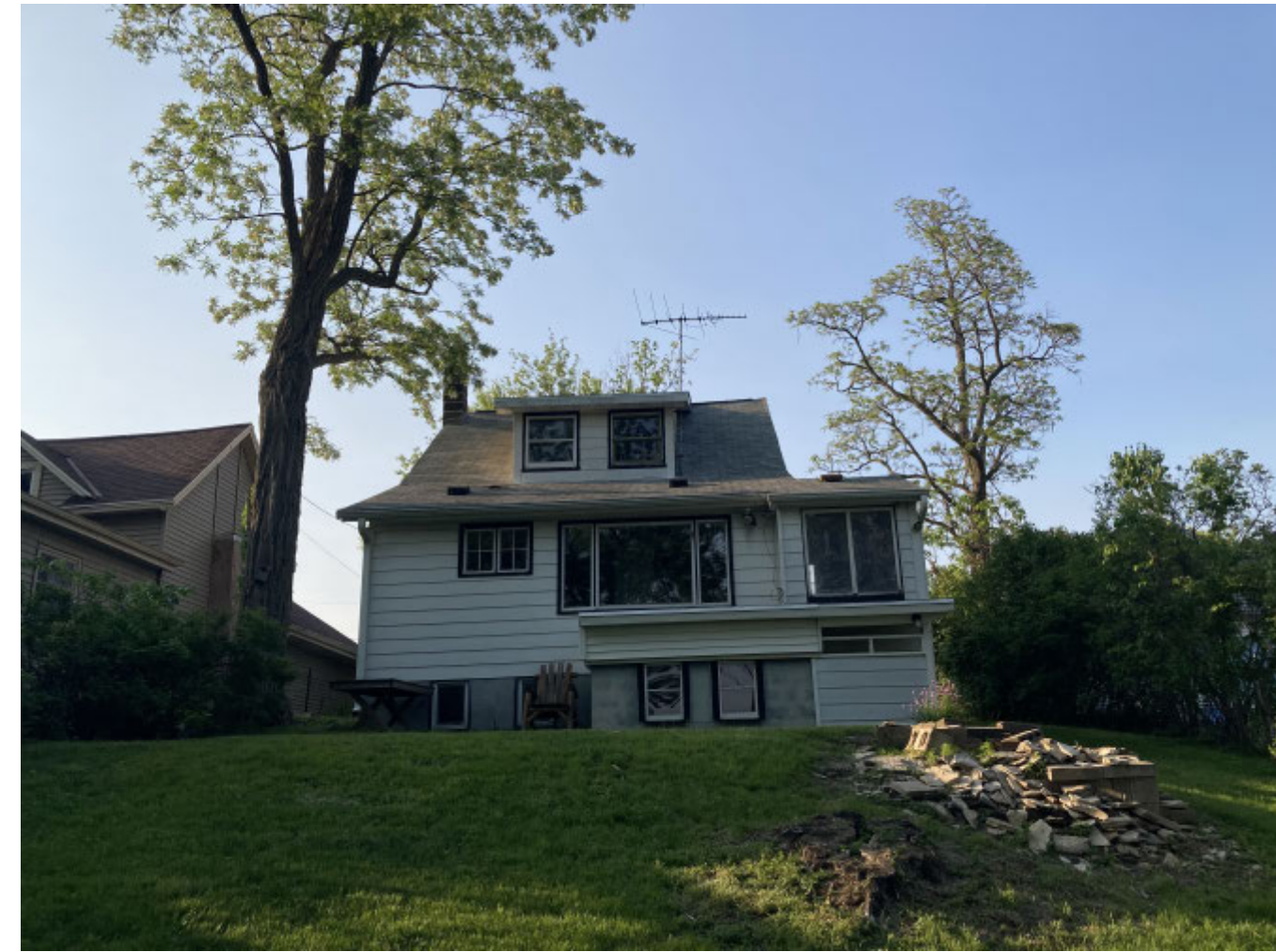
15 EXISTING EXTERIOR PHOTO - 5 3/8" = 1'-0"
