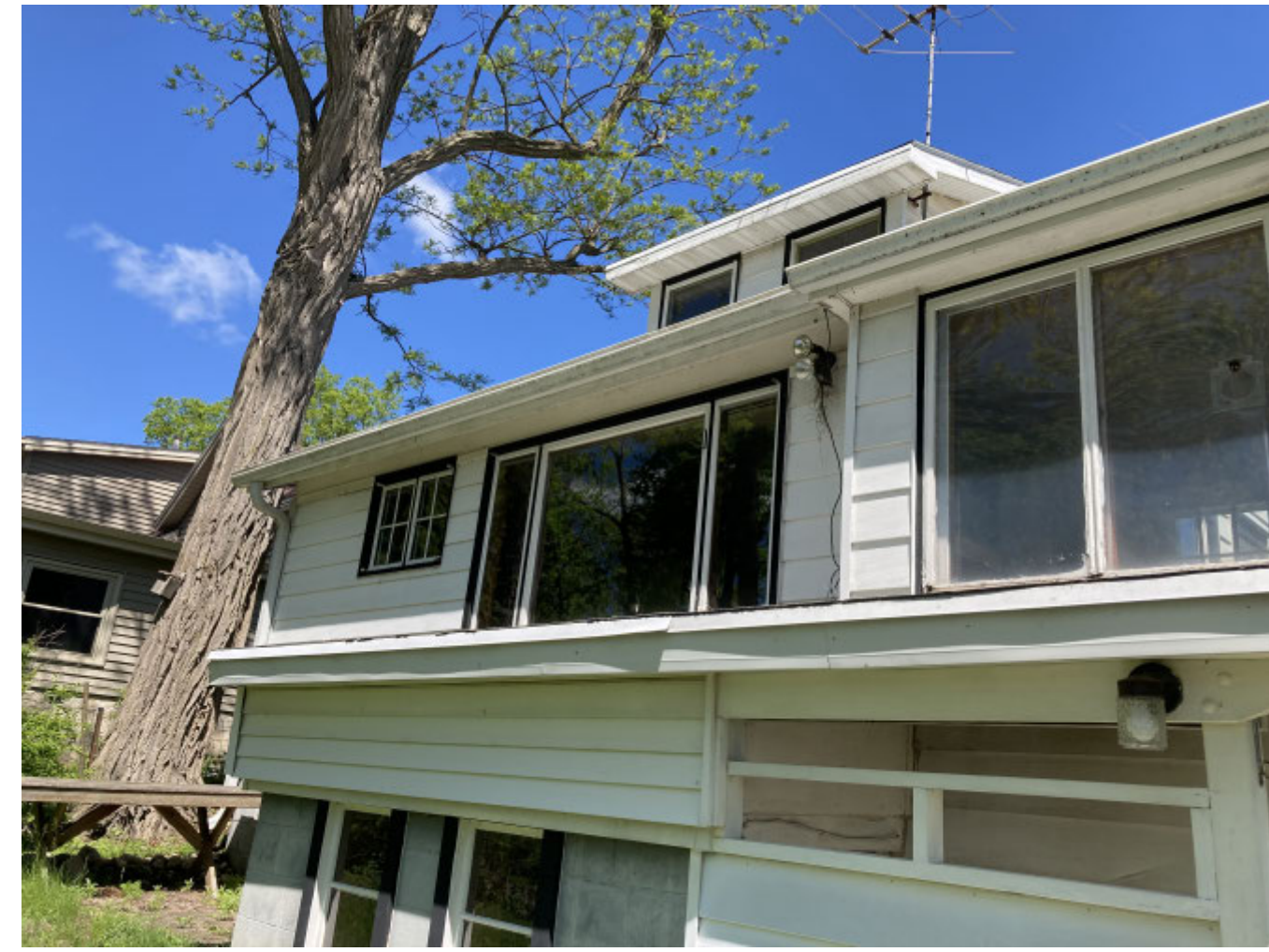
3 EXISTING EXTERIOR PHOTO - 2 3/8" = 1'-0"
