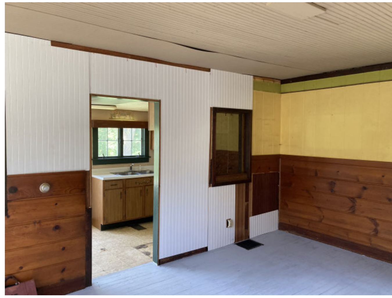
1 EXISTING 1ST FLOOR PHOTO - 1 3/8" = 1'-0"
