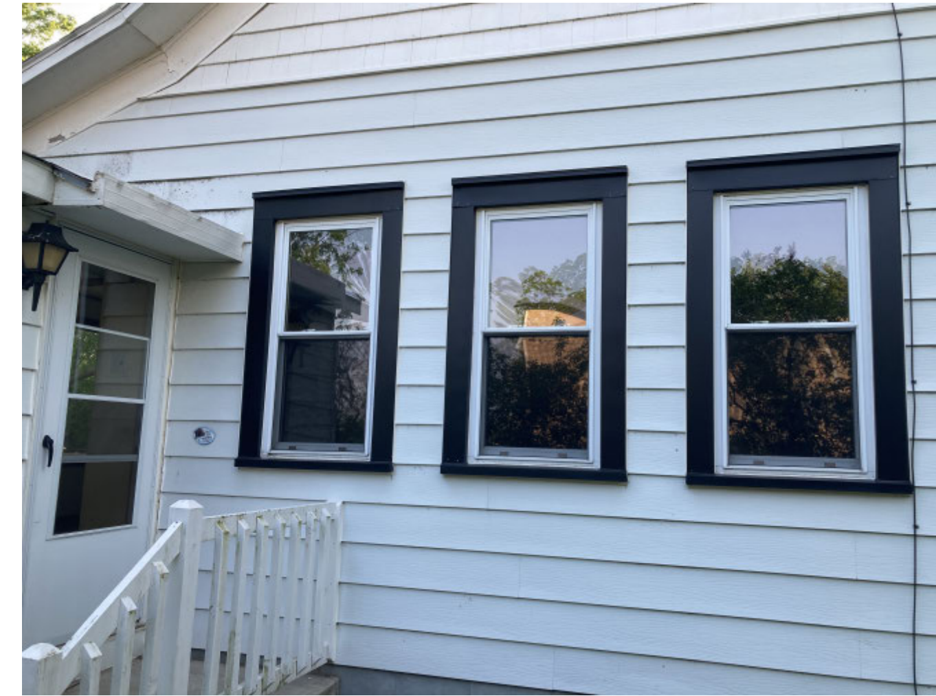
17 EXISTING EXTERIOR PHOTO - 6 3/8" = 1'-0"
