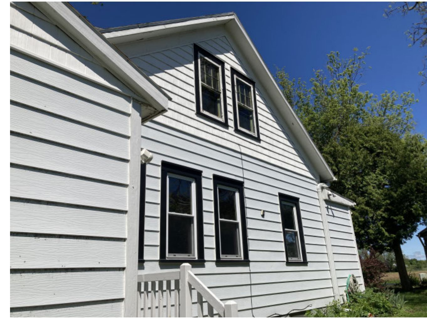
5 EXISTING EXTERIOR PHOTO - 3 3/8" = 1'-0"
