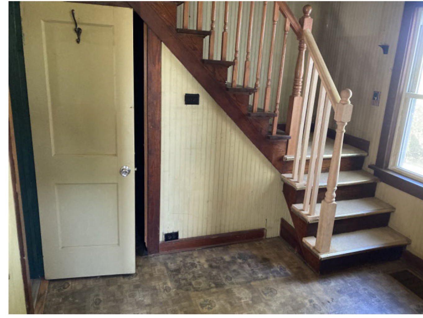
2 EXISTING 1ST FLOOR PHOTO - 2 3/8" = 1'-0"
