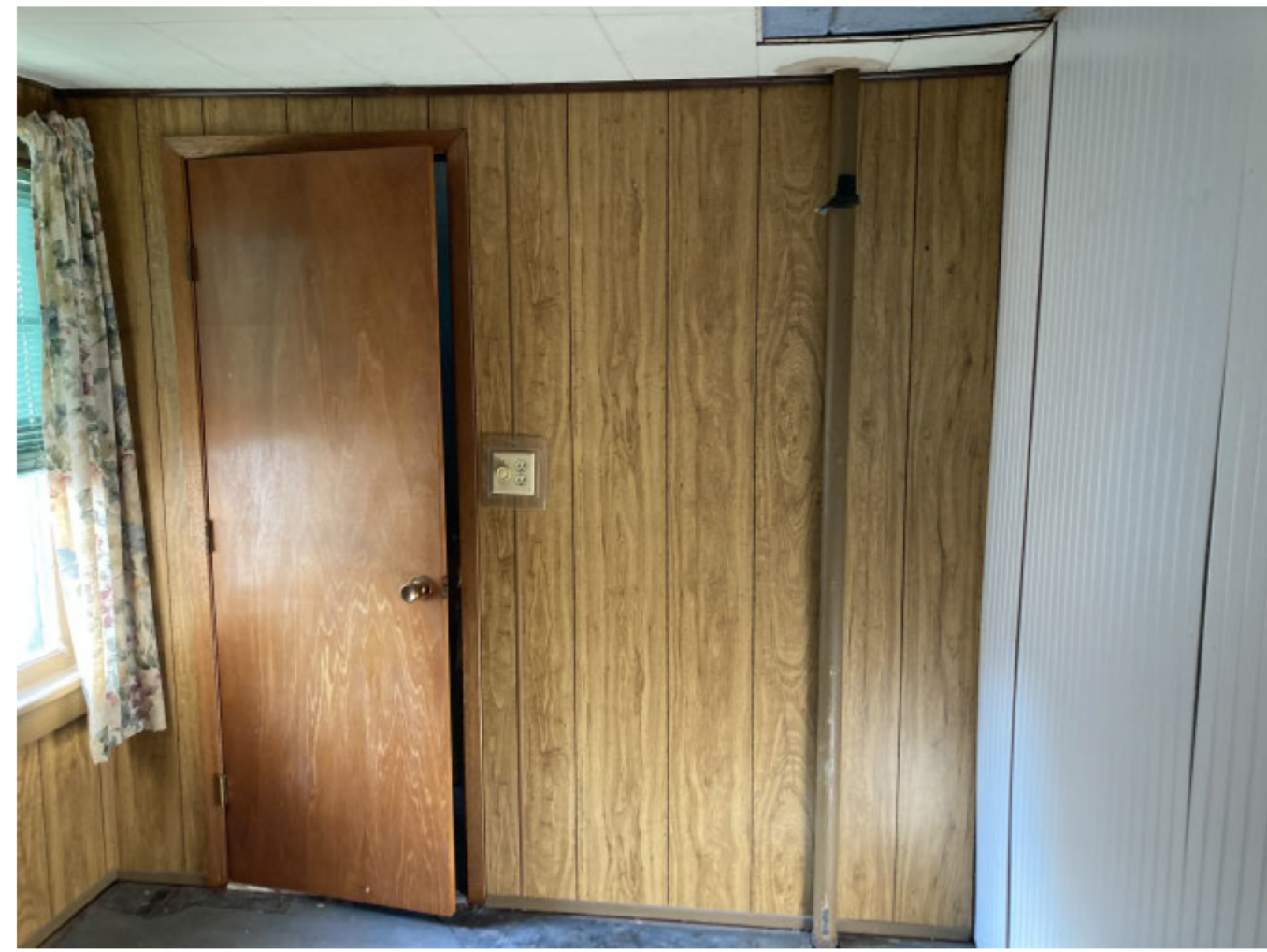
2 EXISTING 2ND FLOOR PHOTO - 2 3/8" = 1'-0"
