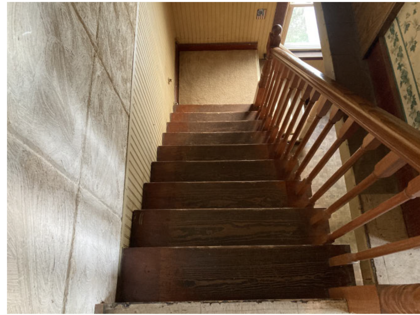
3 EXISTING 2ND FLOOR PHOTO - 3 3/8" = 1'-0"
