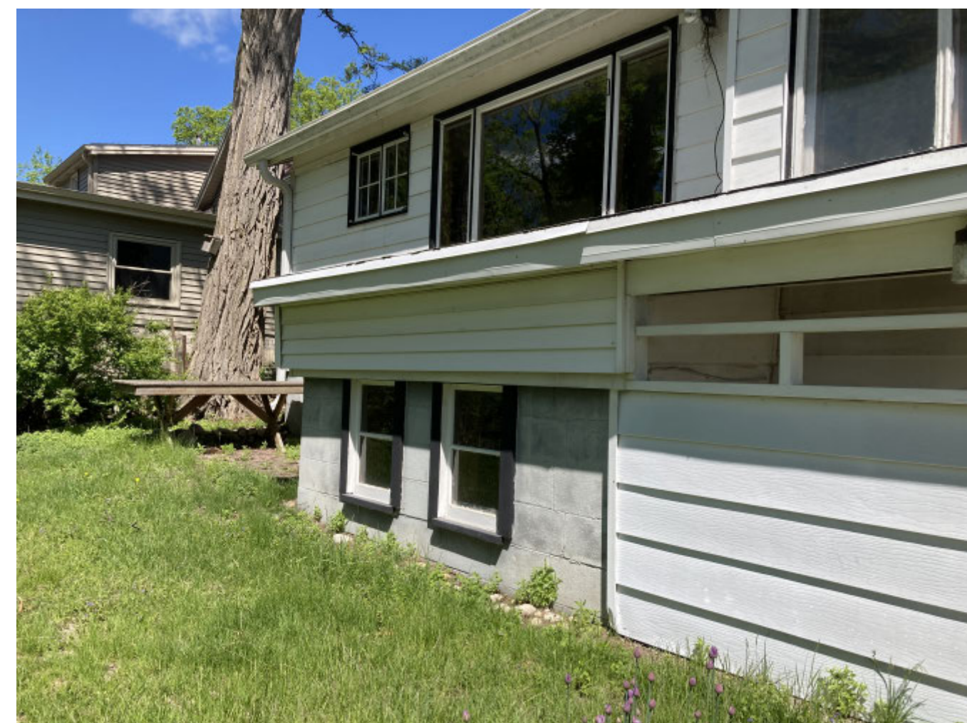
21 EXISTING EXTERIOR PHOTO - 8 3/8" = 1'-0"
