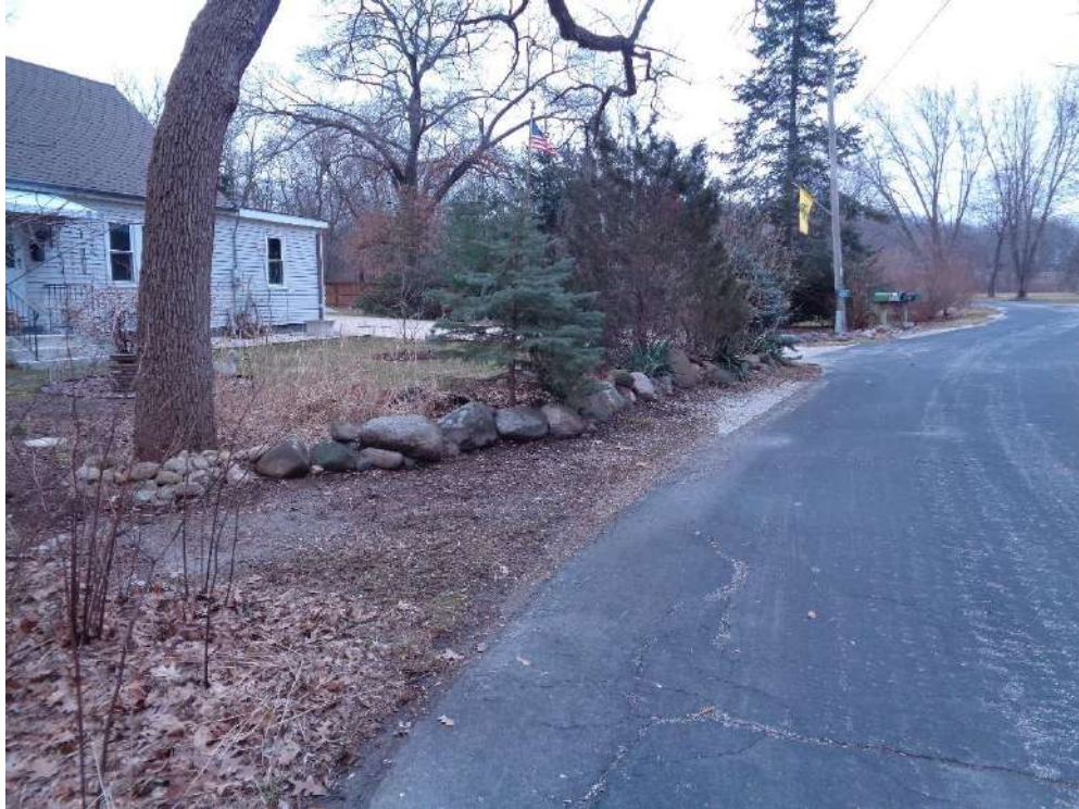
Facing south, just north of property line depicting ROW in front of 1920 N Oak Grove Rd
