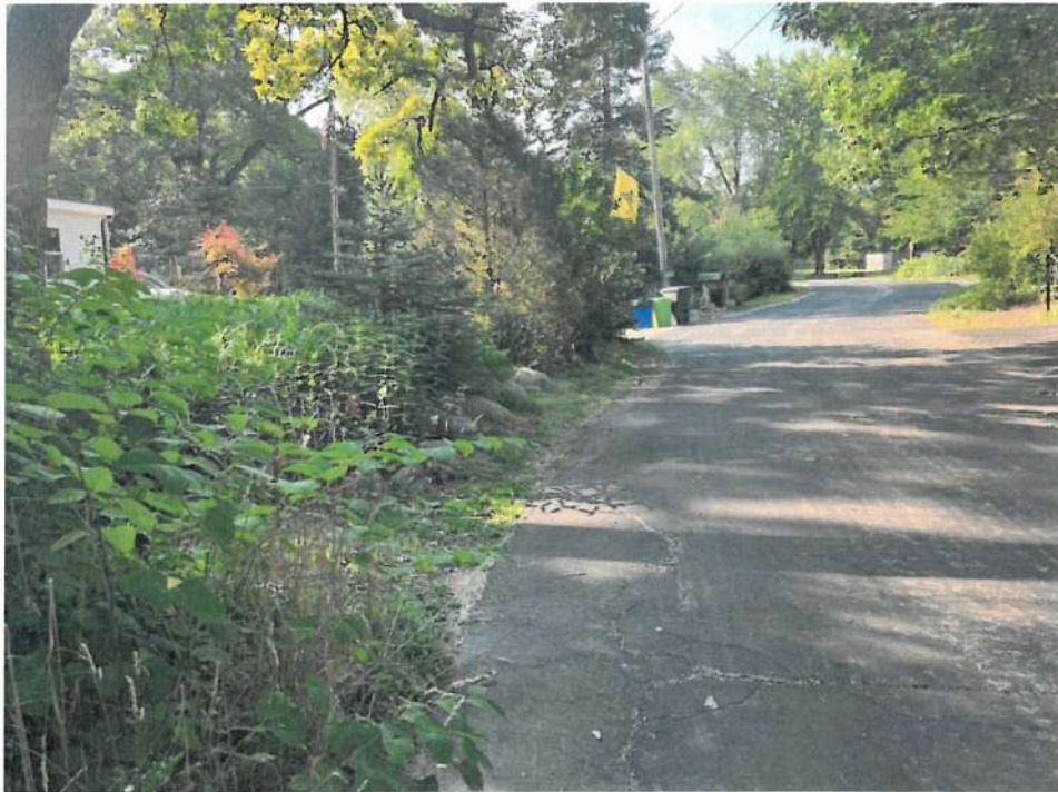
Image of Obstructions and Encroachment of Public Right-of-Way
