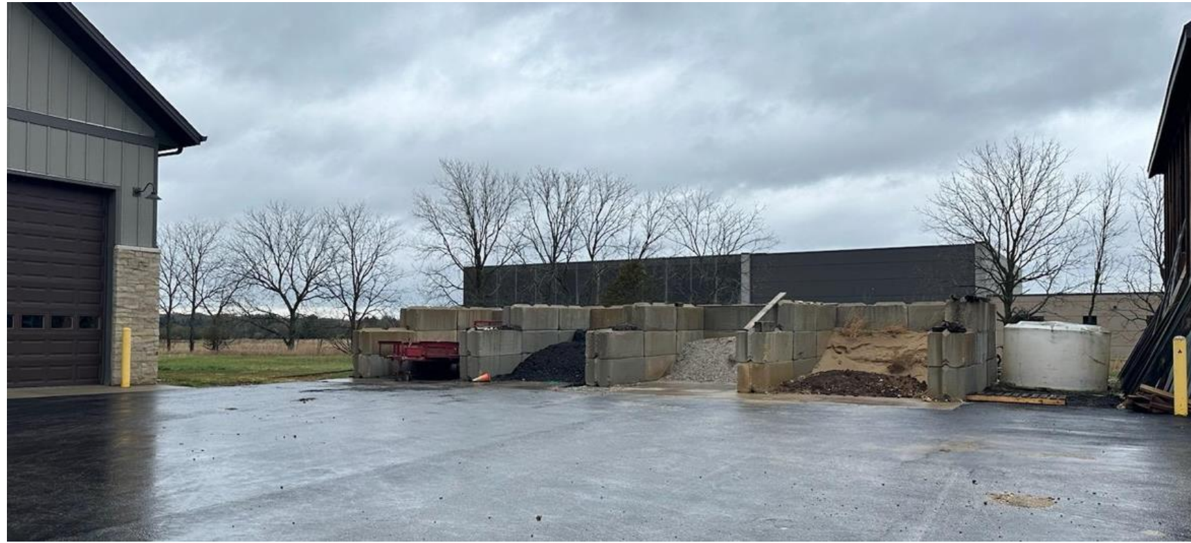
Landscape Basins between Salt Shed & DPW Building (concrete full block construction, 6' height at rear wall)
