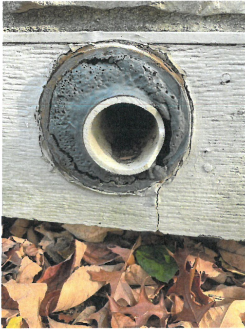
Photo 3 Lift Station No. 3: Baseboard trim damages.
