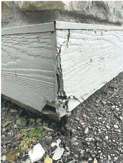
Photo 3 Lift Station No. 3: Baseboard trim damages.
