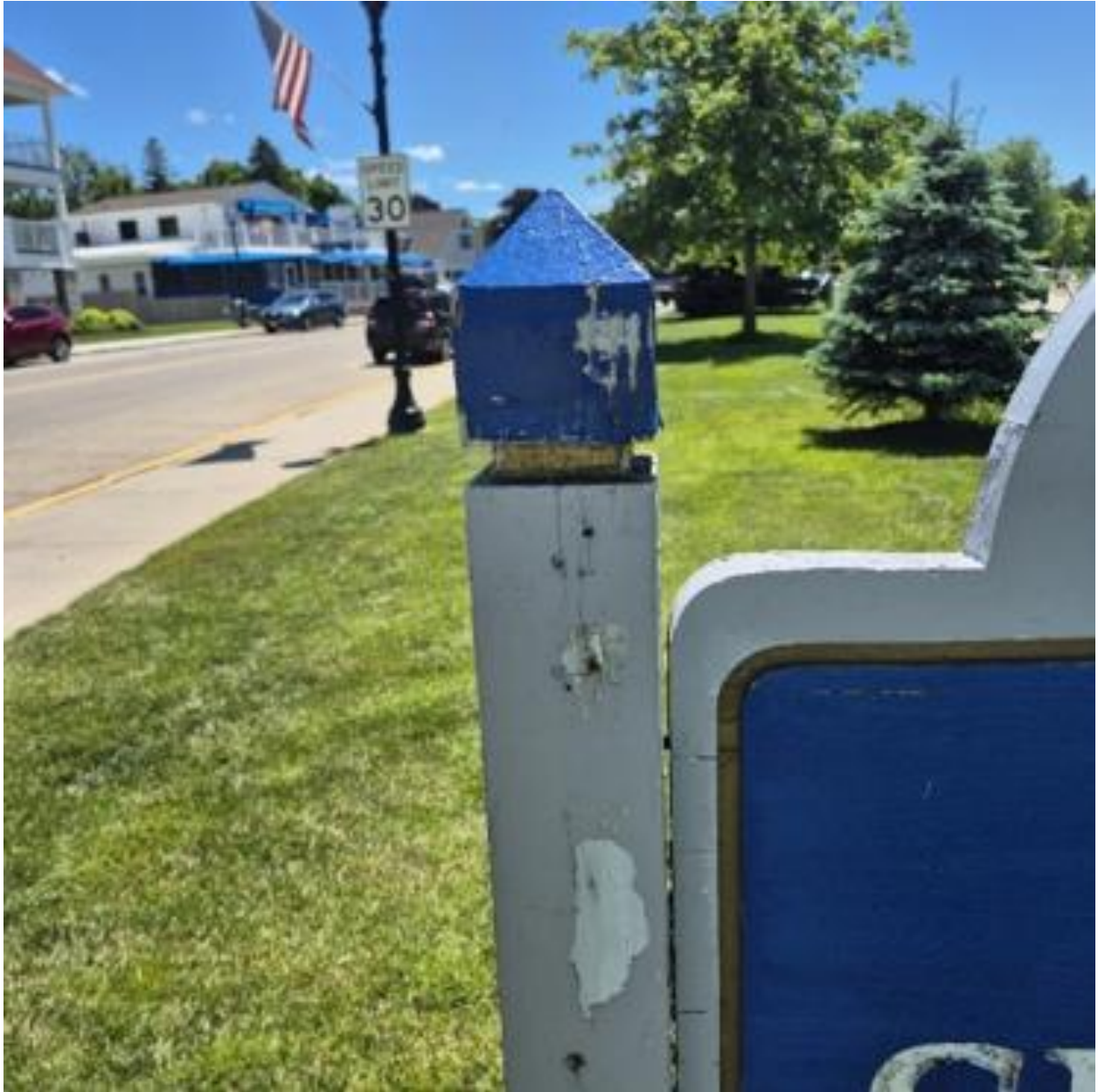
Figure(s) 3 - Sign Deterioration
