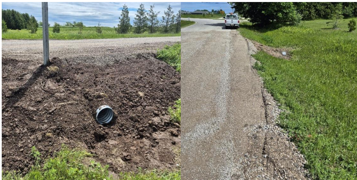
Figure(s) 1 - Orchard Drive; Culverts
