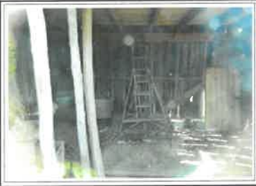
Interior of Storage Shed
