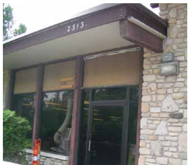
Park Maintenance Building
