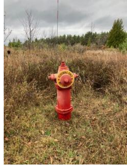
Picture 1.3 – Hydrant 254 was classified as a flushing only hydrant, not for fire flow due to low residual pressure while performing fire flow tests.
