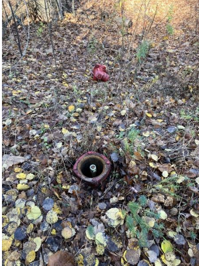
Picture 1.1 – Hydrant on Maple Drive that was hit and was reported by a pedestrian walking by who noticed the damage.
