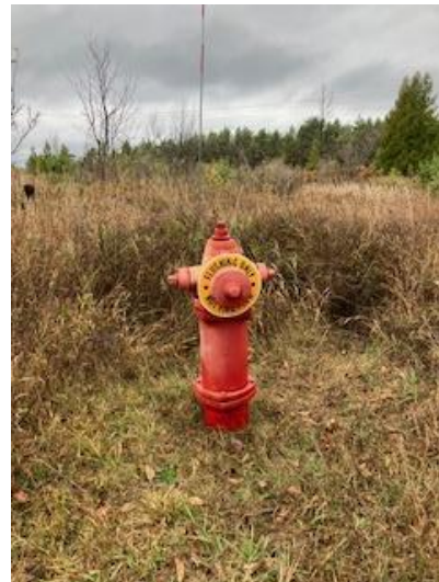
Picture 1.3 – Hydrant 254 was classified as a flushing only hydrant, not for fire flow due to low residual pressure while performing fire flow tests.
