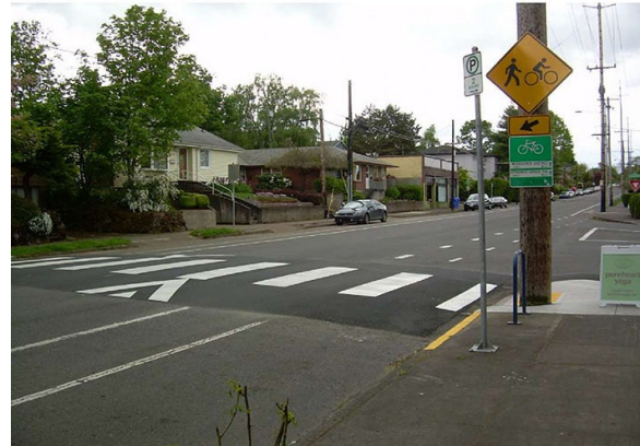
Raised Crosswalk Example
