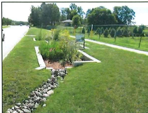
Example of a bioretention system designed to treat stormwater and protect adjoining surface waters
