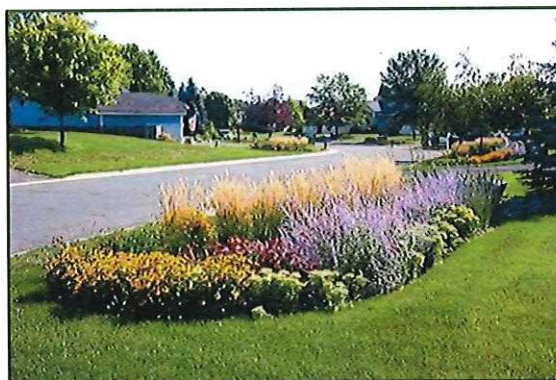
Example of LID system designed to treat residential runoff, courtesy Thurston Regional Planning Council
