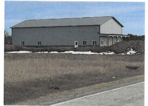
27. 5000sf JF Construction Cty ZZ
