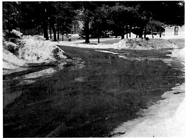
As spring thaw weakens pavements, trucks carrying heavy loads can damage them.
