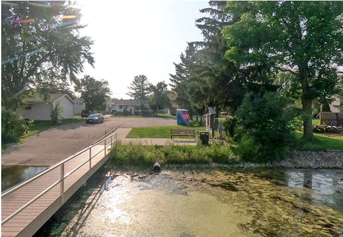
Black Otter Lake - Shadow Boat Launch Storm Outfall - Looking West
