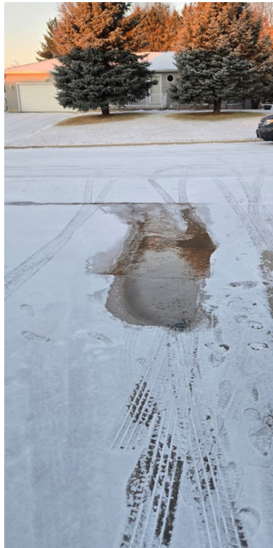
Figure 2: Photo of water leak on Birch Street
