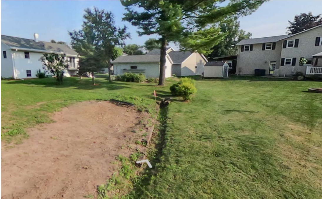
Drainage Easement- Inlet Pipe Near 229 Lakeshore Drive – Looking South
