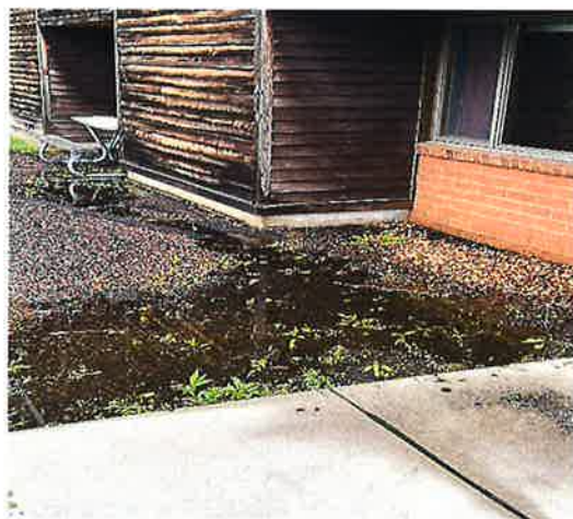
TAGS: Landscaping COMMENTS: Photo taken 5 hours after rainstorm ponding issues
