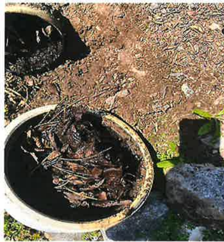
TAGS: Landscaping COMMENTS: Plugged cap from collector
