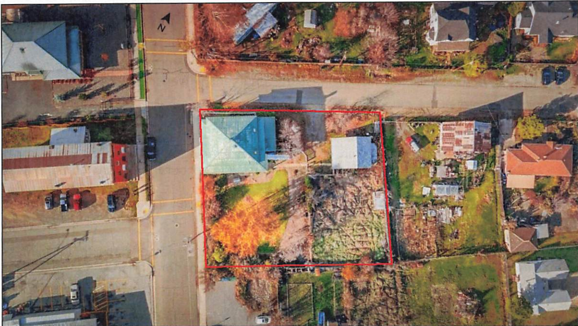
Figure 3, Project Site Aerial Overview (parcel boundaries are approximate)
