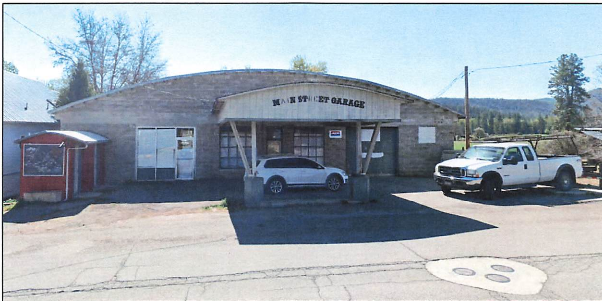
Figure 2, 504 Main Street (facing south)
