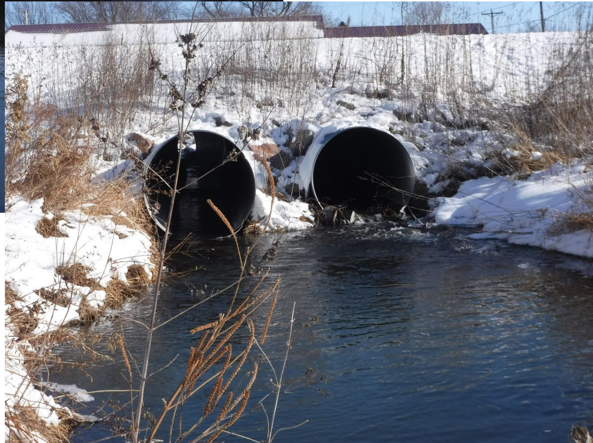
72" CMP Culverts at RR Grade
