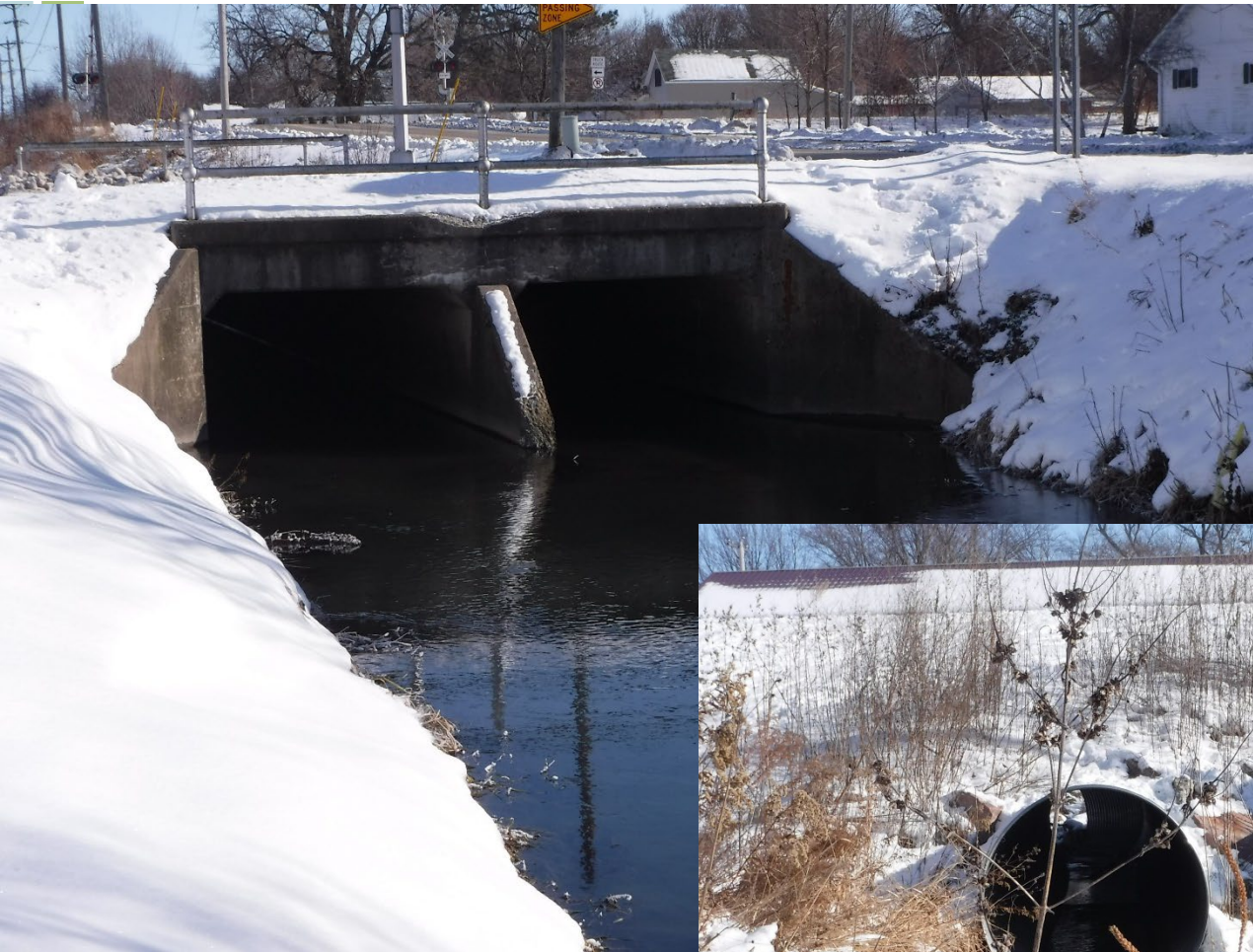
10'W x 6'D RCBC at Aspen Ave
