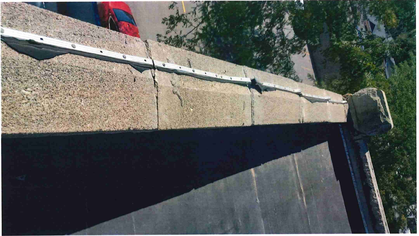
Pics showing Failed Corner Flashing and detached Field Membrane:
