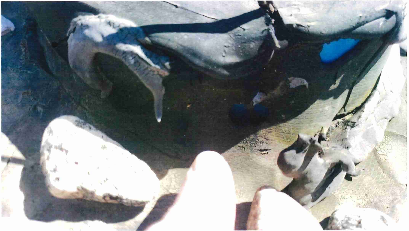
Holes in Exhaust Curb Corners:
