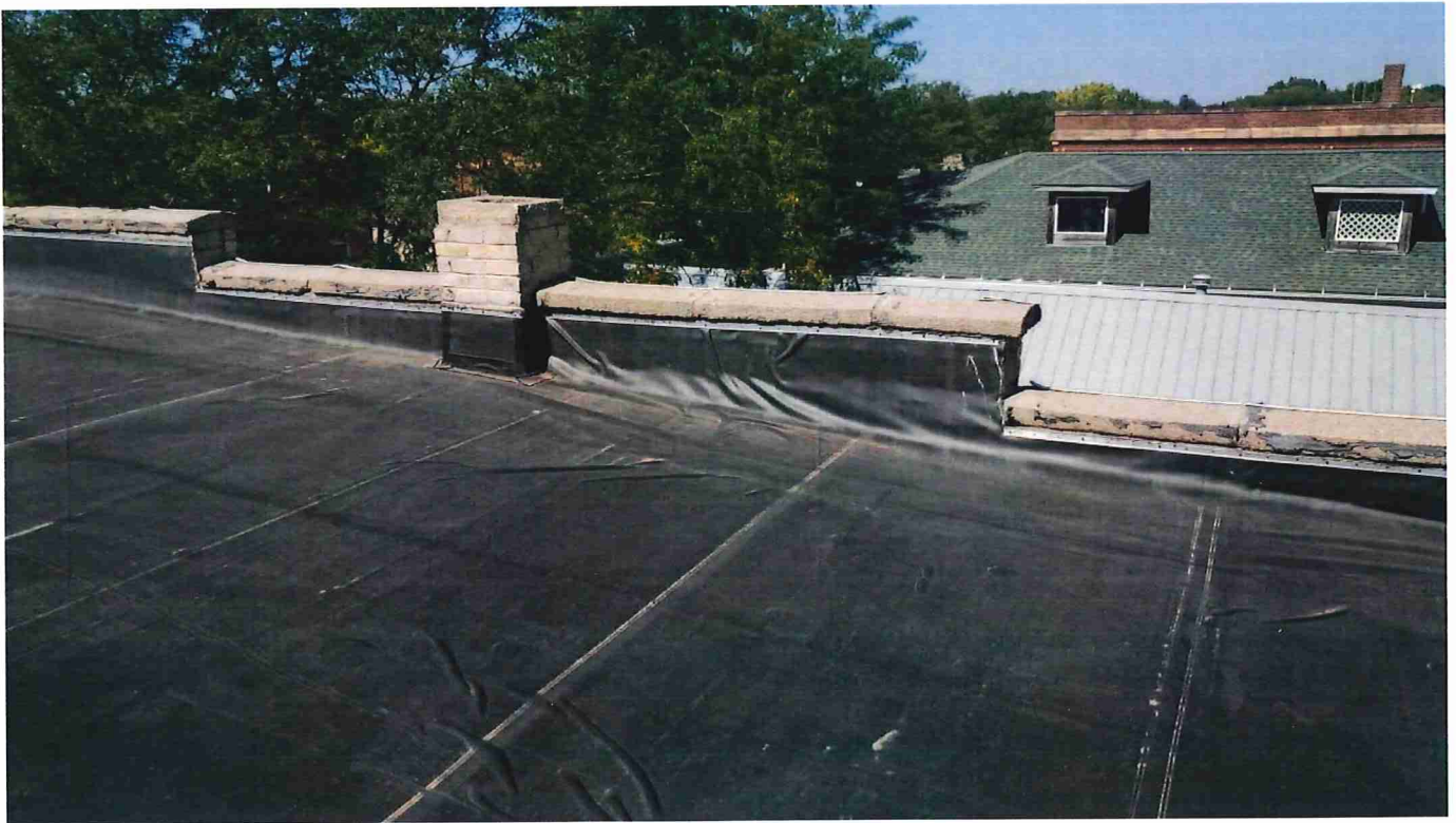
Pics showing Failed Corner Flashing and detached Field Membrane:
