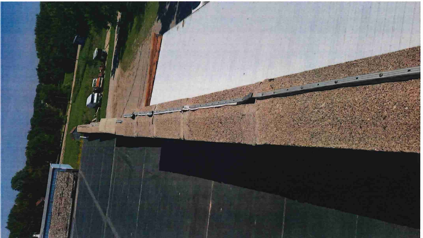
Pics showing Old termination bar left on walls from previous contractor/installer:
