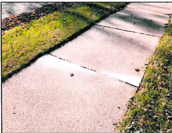
Sample Repair Photo: Defect 30 repaired on 11/03/25 at 242 Wood Ave at 12:56 PM
