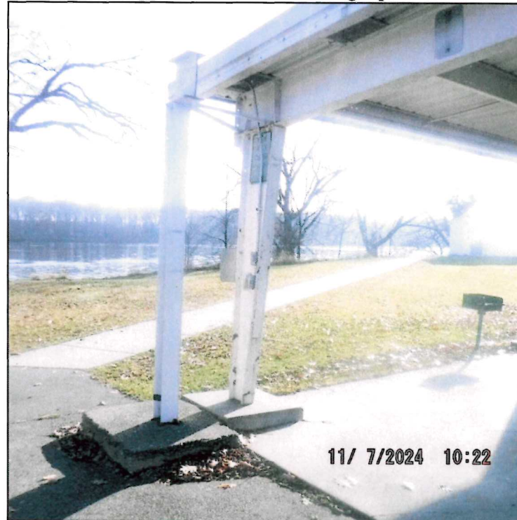
Figure 2. Typical raised pier foundations (Northernmost piers).
