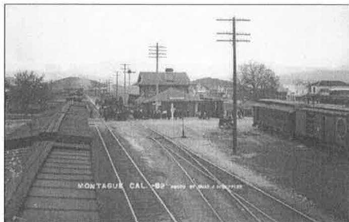
Figure 2-1, Montague Train Depot (1912)
