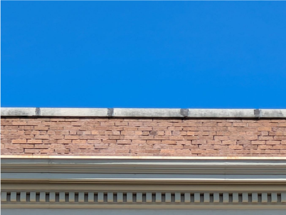
East facing façade.
