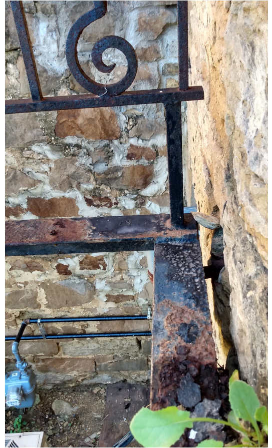
West angle iron ledger bolt has also moved away from the wall ~1.3 inches.
