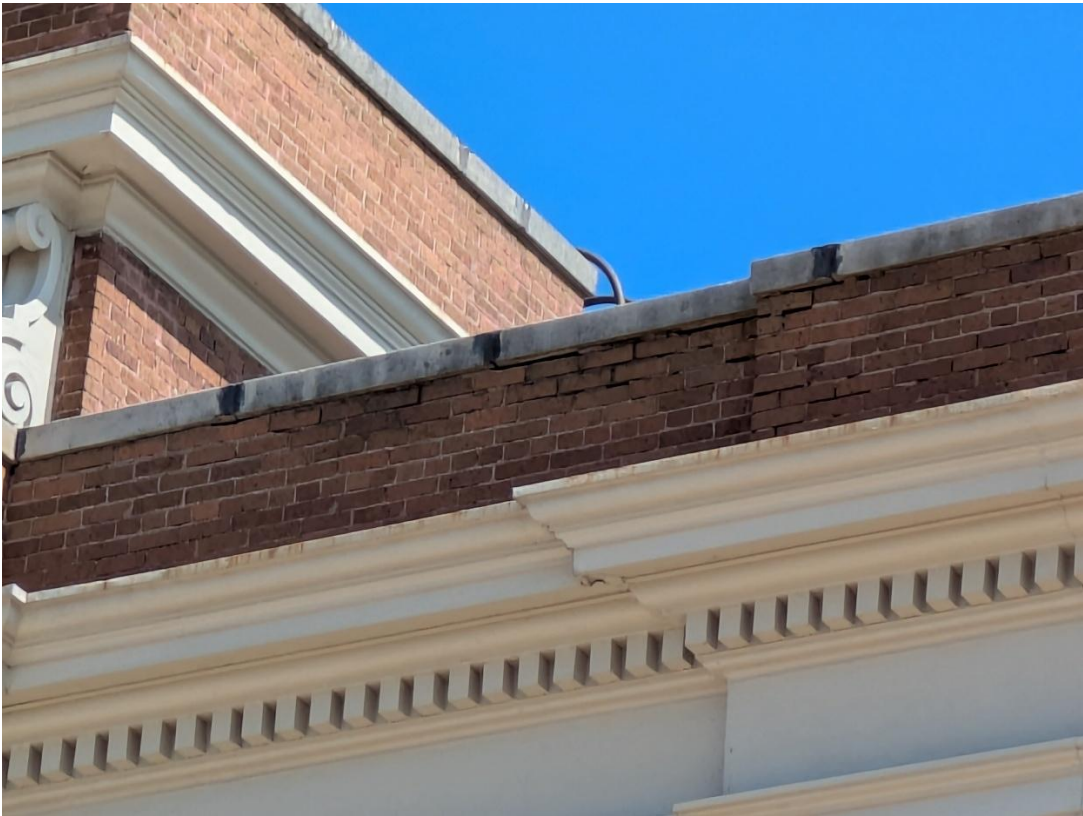
South Facing Façade.
