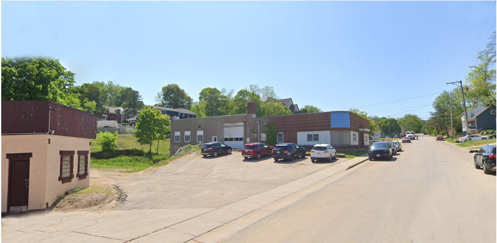
Existing View from Northeast
