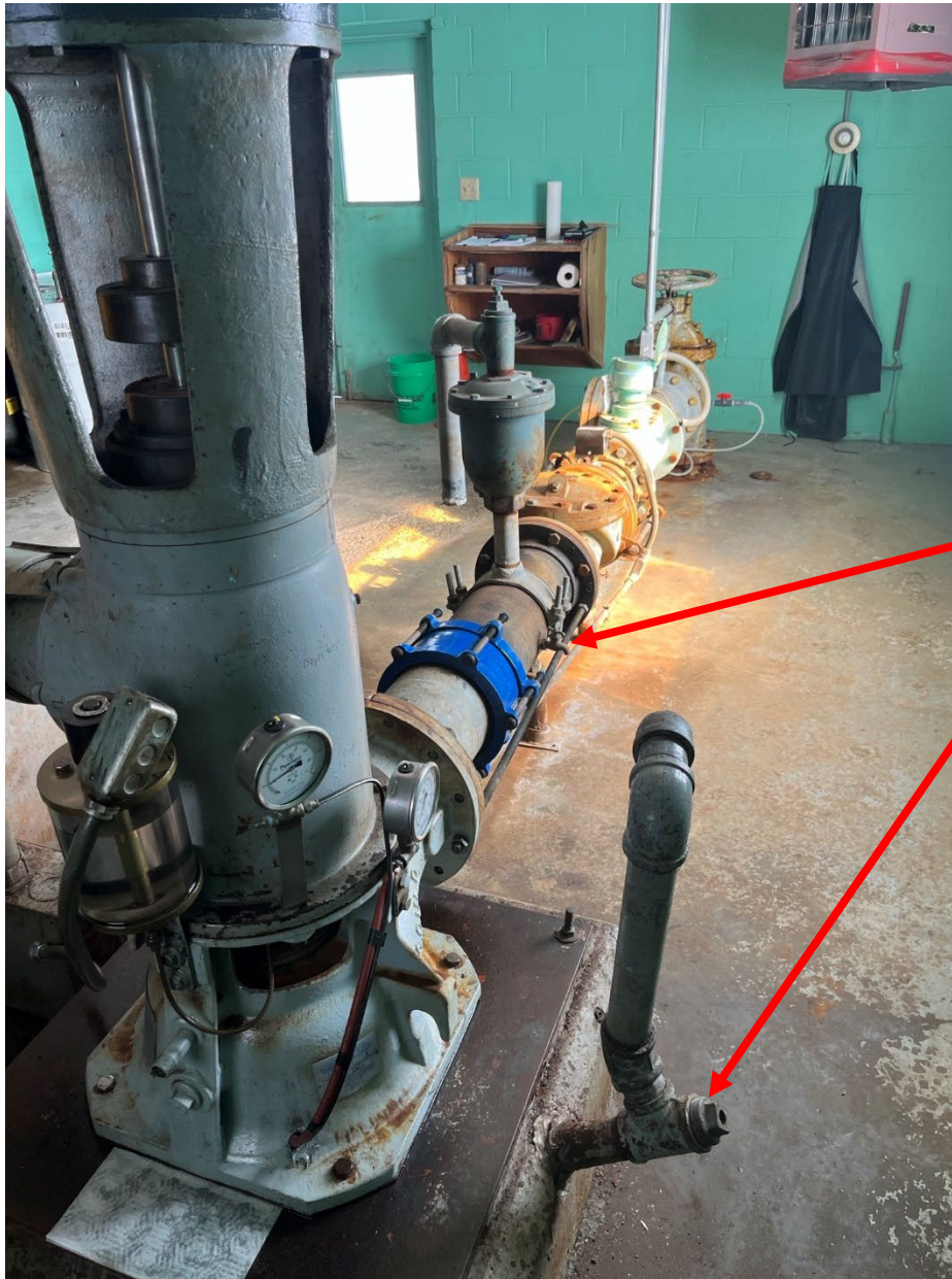
Figure 2. Well water recycle line connection detail/well water recycle line connection detail with existing sample tap.
