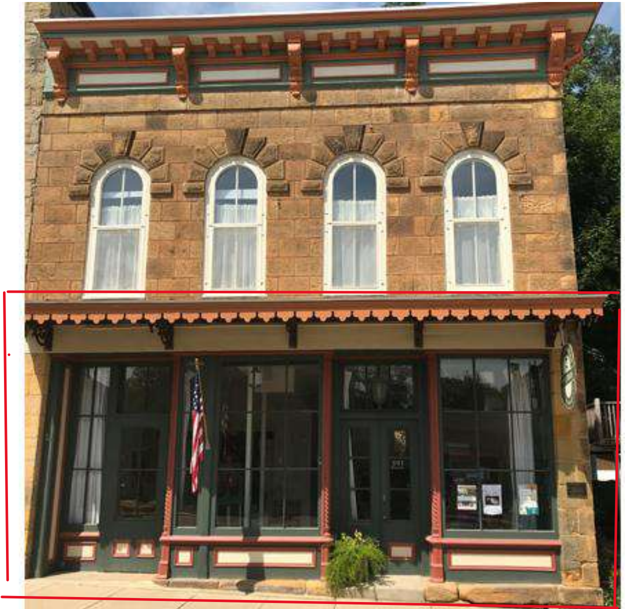
Façade, view from across High Street. Area of proposed work indicated.
