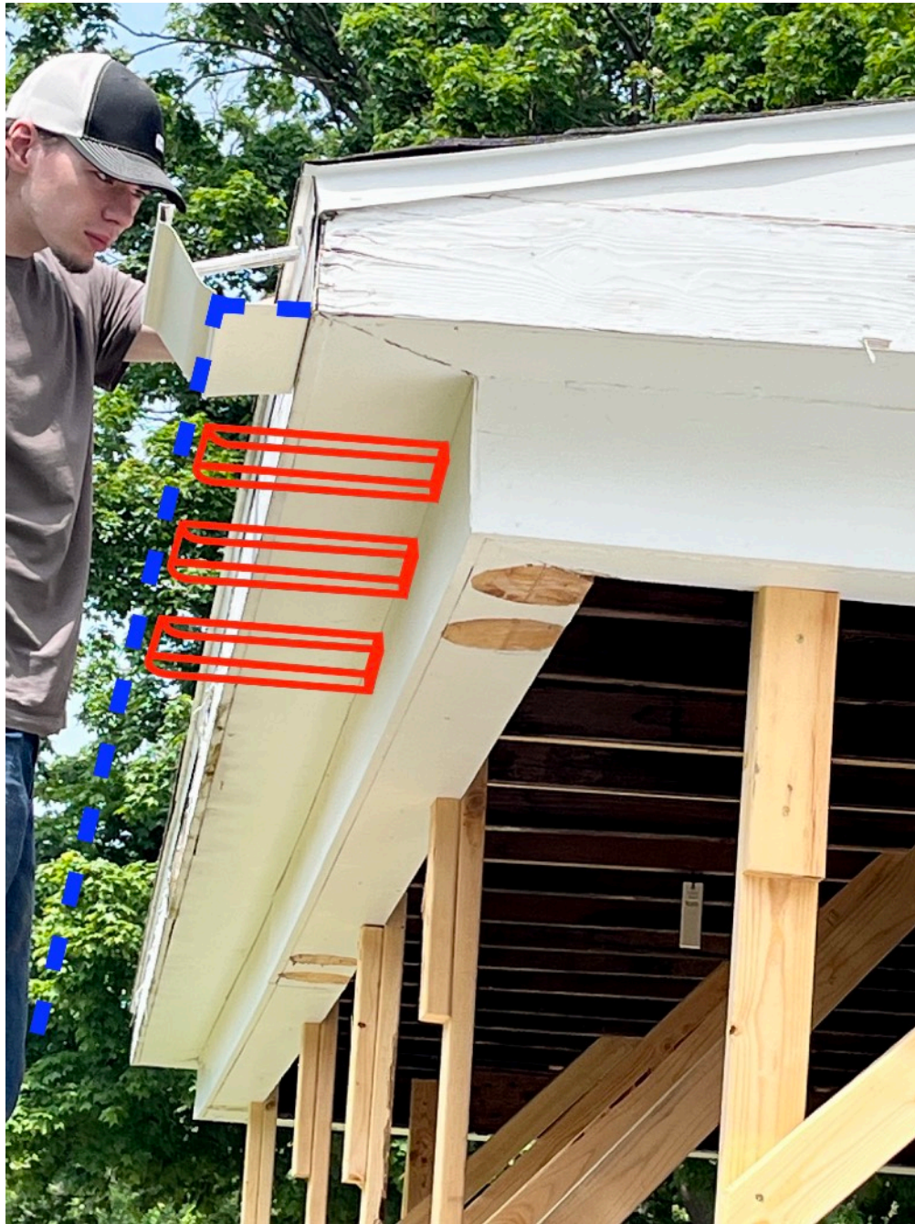
Porch K-style gutter, with dentil corbel added underneath eave
