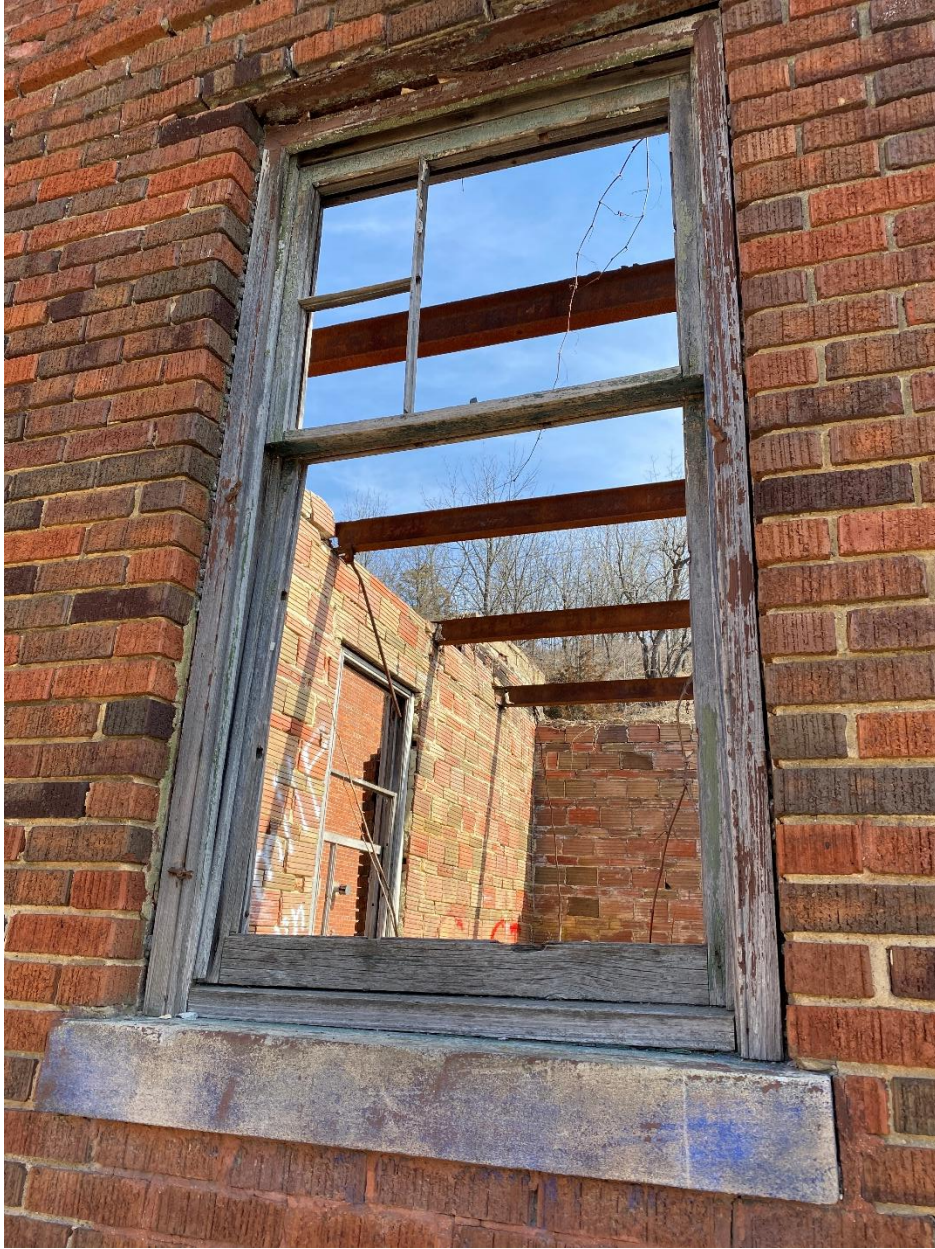
Roof steel condition as seen from the west
